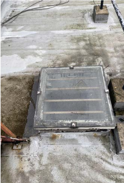
Typical existing roof light proposed to be replaced
