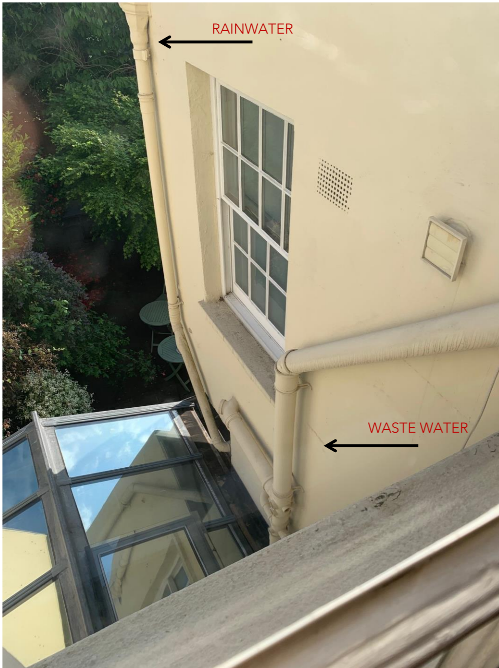
EXISTING PHOTOGRAPH OF REAR ELEVATION FROM FIRST FLOOR WINDOW
