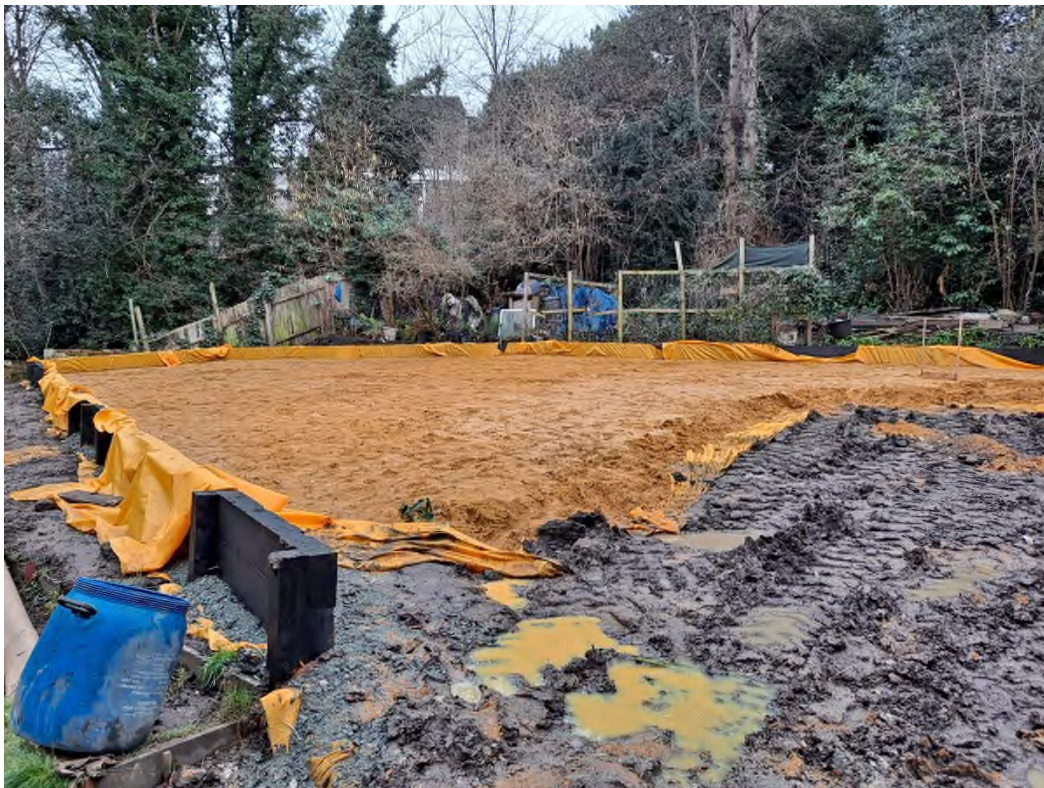
Plate 6: VISIT 15/02/22 – Laying of subsoil over membrane in the location of former plots 29 and 30 (northwest of site)
