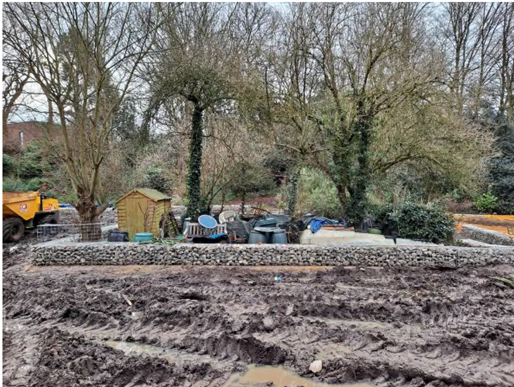
Plate 2: VISIT 15/02/22 – Gabion constructed around the communal area
