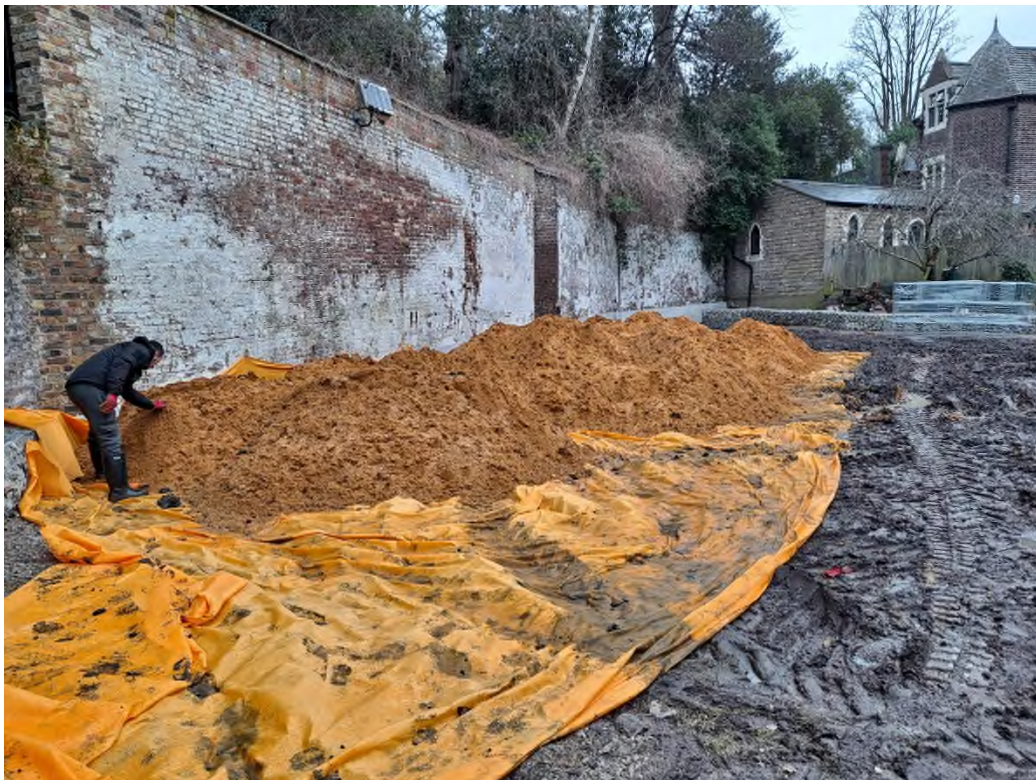
Plate 4: VISIT 15/02/22 – Subsoil stockpiled on membrane in north of site
