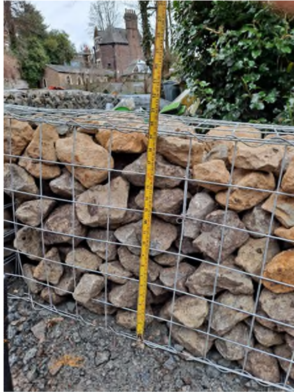
Plate 3: VISIT 15/02/22 – Confirmation of Gabion height – 500mm
