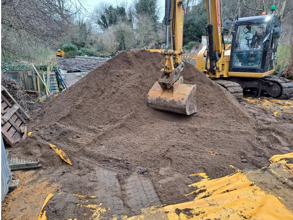
Plate 5: VISIT 15/02/22 – Topsoil stockpiled on membrane adjacent to the site entrance
