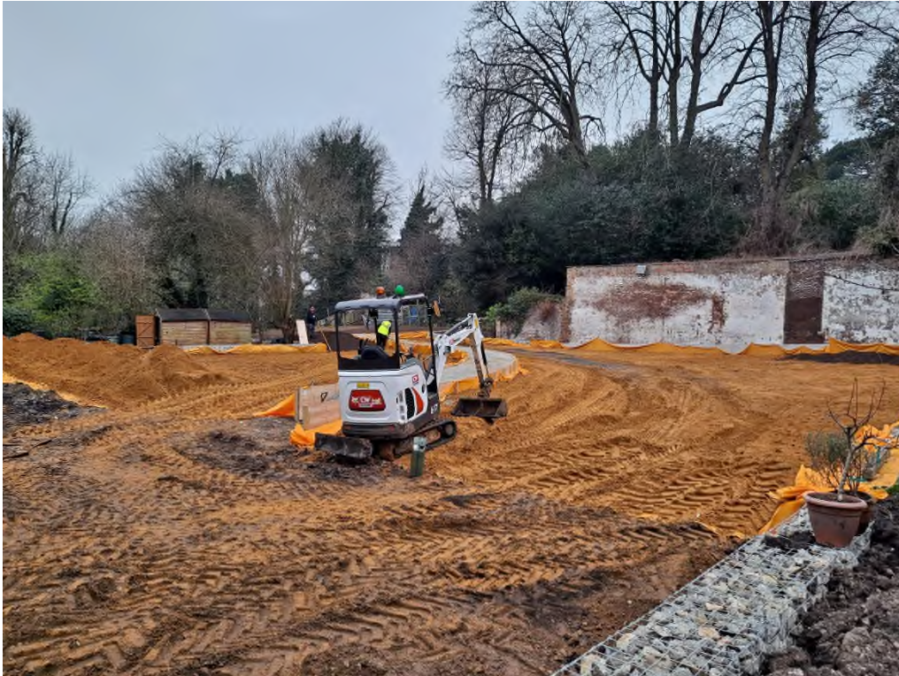
Plate 11: VISIT 16/03/22 – central region of the site: membrane and subsoil placed, topsoil being placed (behind the excavator)
