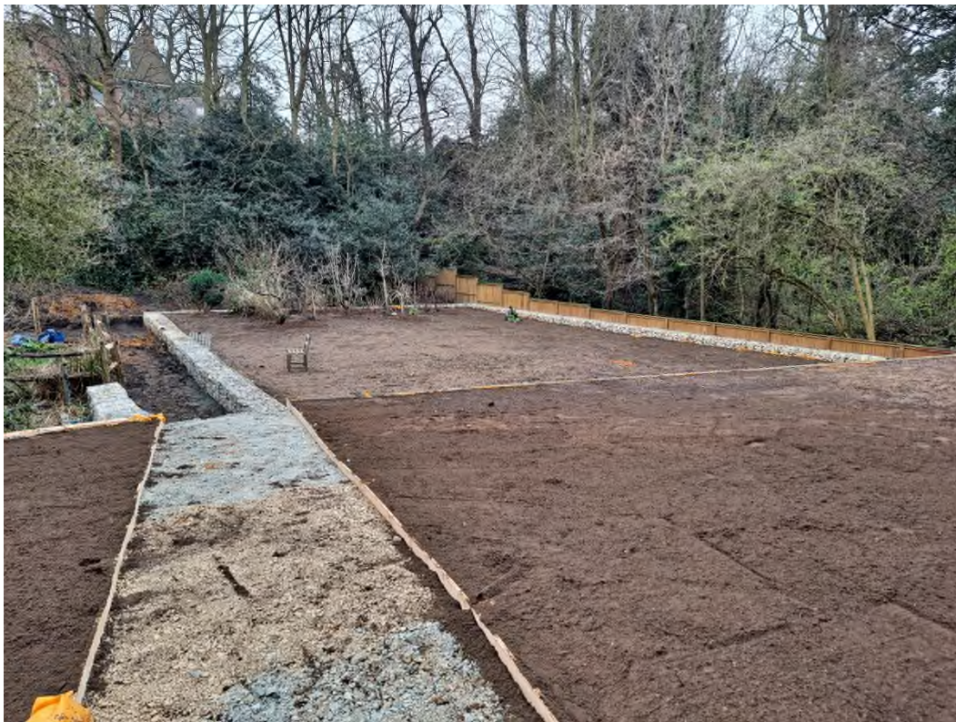
Plate 10: VISIT 16/03/22 – rear (west) of the site with placement of clean cover soils completed
