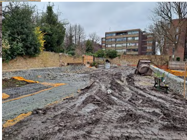
Plate 2: VISIT 15/02/22 – Gabions under construction in the northern regions of the site
