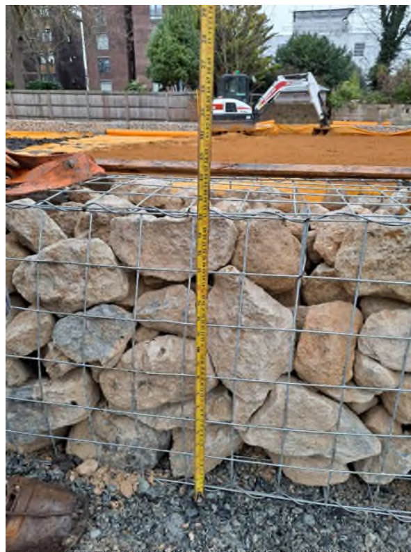
Plate 4: VISIT 15/02/22 – Confirmation of Gabion height – 500mm
