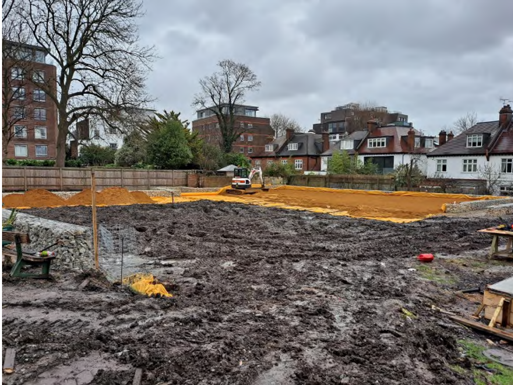
Plate 3: VISIT 15/02/22 – View looking east showing subsoil application over membrane in the southeast of the site
