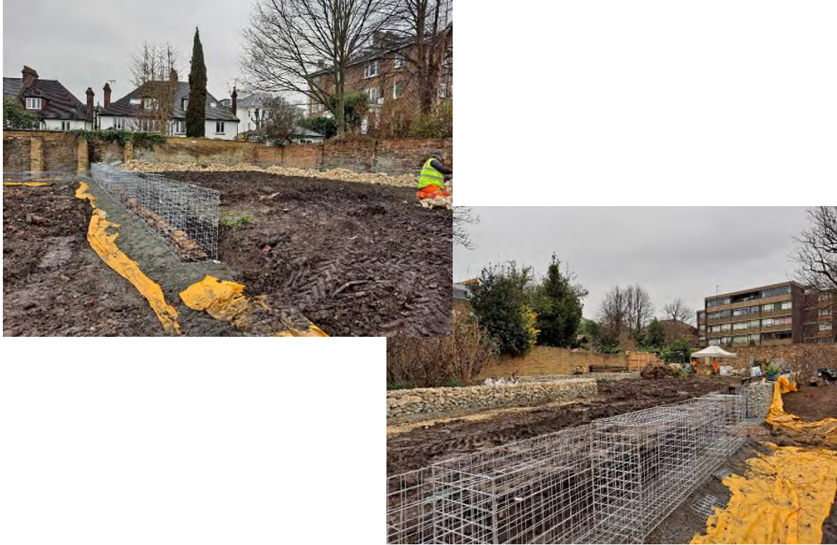
Plate 11: VISIT 16/03/22 – Gabion wall construction at the rear of the site
