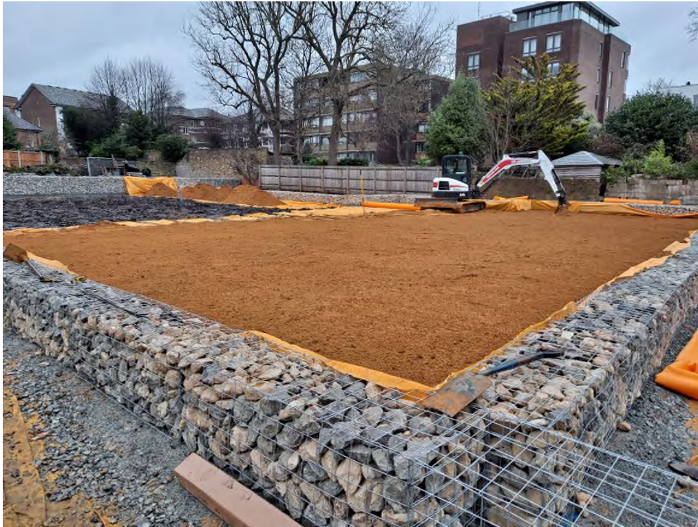
Plate 7: VISIT 15/02/22 – Subsoil being applied over membrane in the southeast of the site. Verification samples taken from this area (#2) and from the stockpile in the background (#2)
