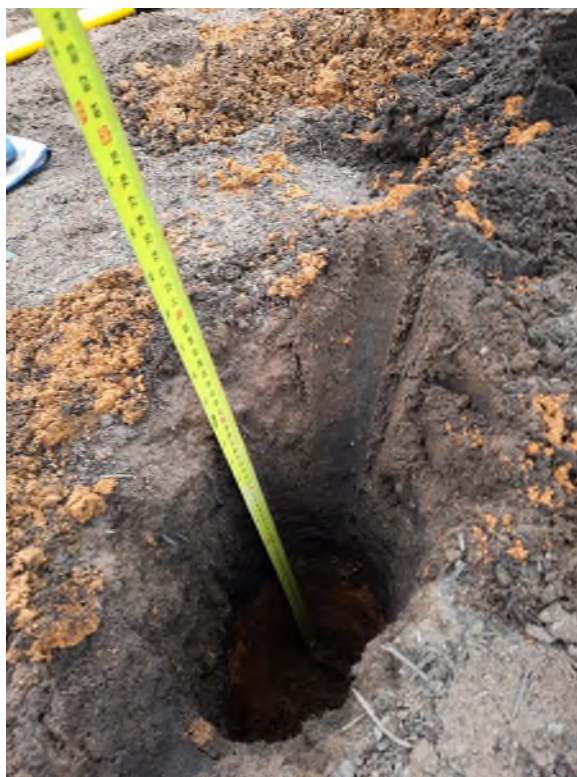
Plate 20: VISIT 05/04/22 – example inspection pit (plot 17b) showing 500mm cover
