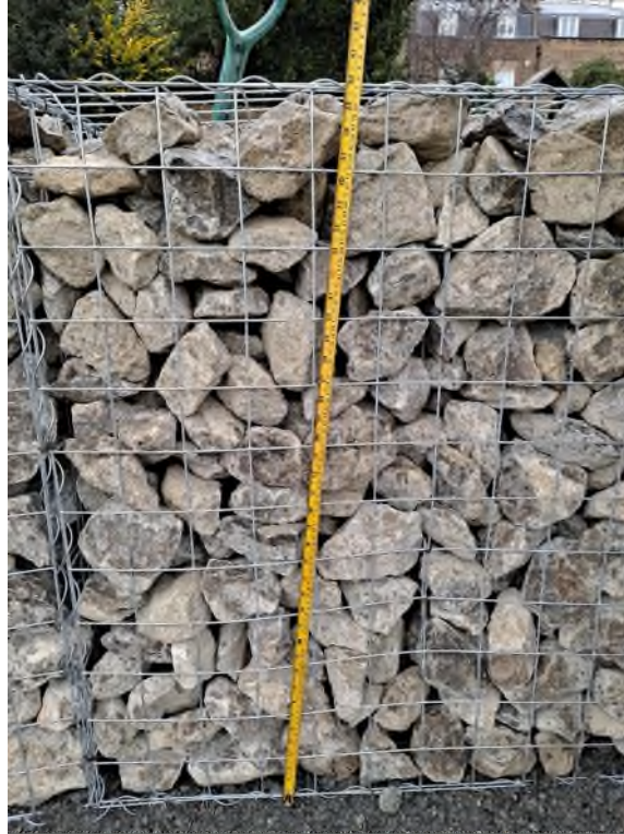
Plate 5: VISIT 15/02/22 – Confirmation of Gabion height in location of former retaining wall – 1,000mm
