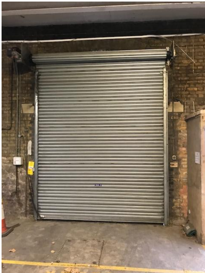
Rear roller shutter door
