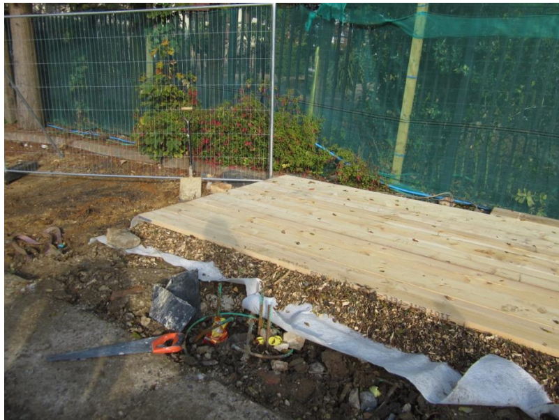
Image 12: Example Temporary Ground Protection - BS5837 - Ground protection, wood chip and scaffold boards: Ground protection incorporating 100mm wood chip layer placed on a geotextile membrane with scaffold board surface to support pedestrian traffic.
