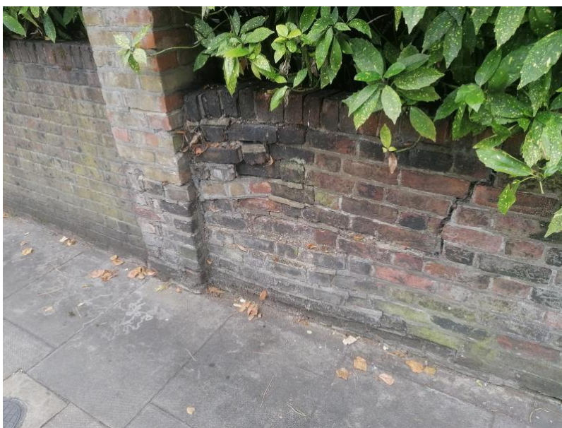
Image 3: damage to wall adjacent to T1.
