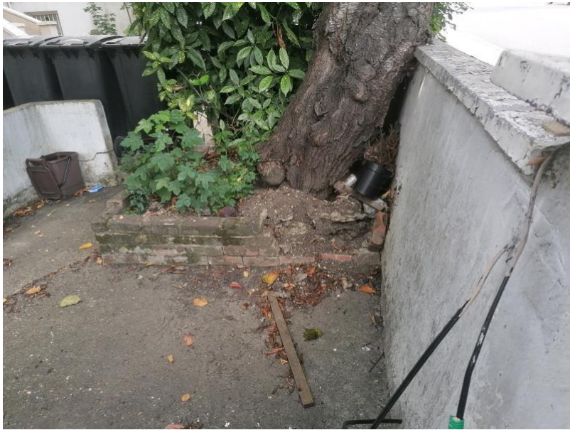
Image 6: hard surfacing around trees will be replaced with porous paving.
