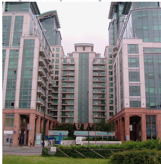
Figure 7: A tunnel effect can occur if a window has projecting wings on both sides of it. In this development in South London (architects Broadway Malyan), the windows have been increased in size to compensate
