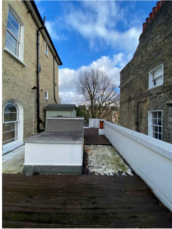
1. Roof of No.4B Looking East
