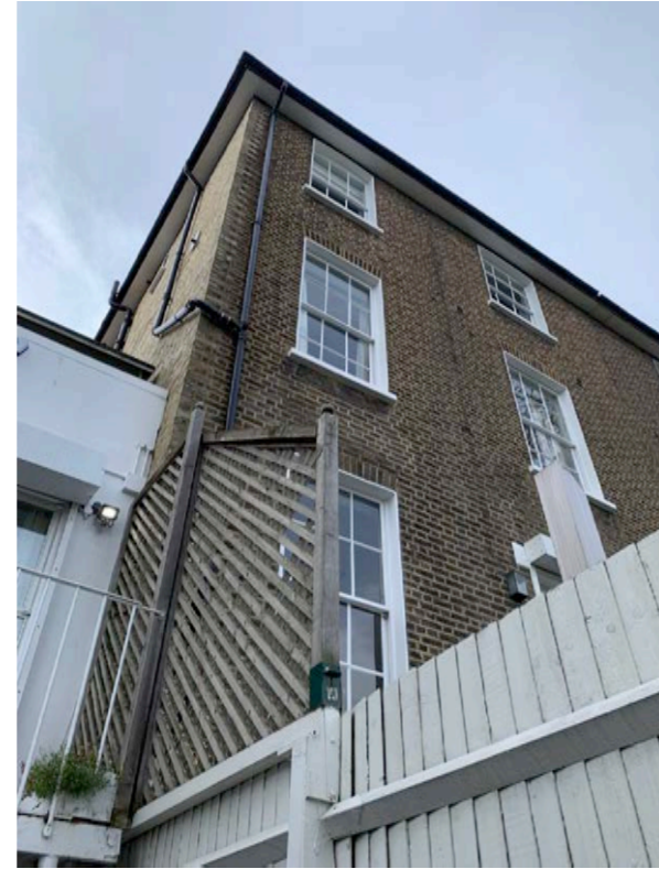
2. Rear of No.4B Looking up at No.4
