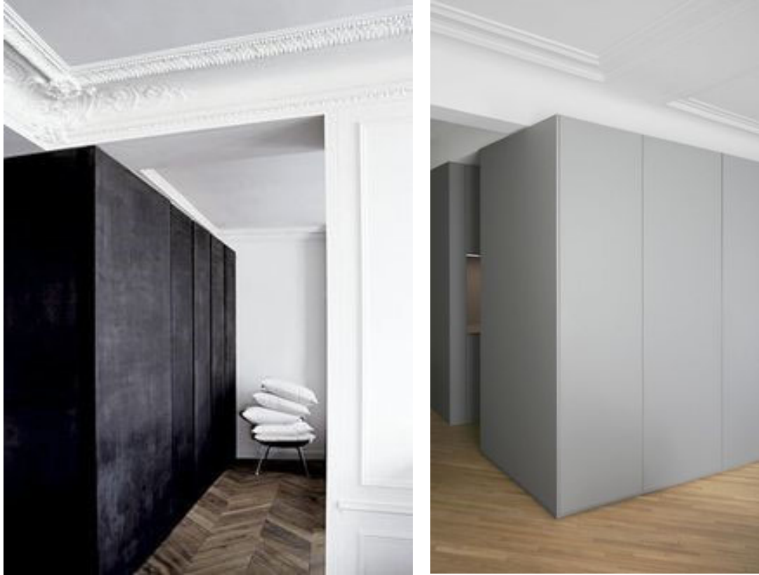
Photograph 2 & 3; examples of similar interventions within clear volumes. Painted panels to pod partitions, shadow 'flash-gap' detail at existing floors and walls.
