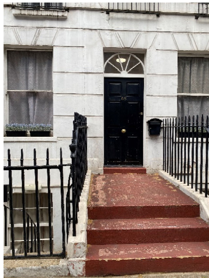
6. Entrance at No65 to be renewed
