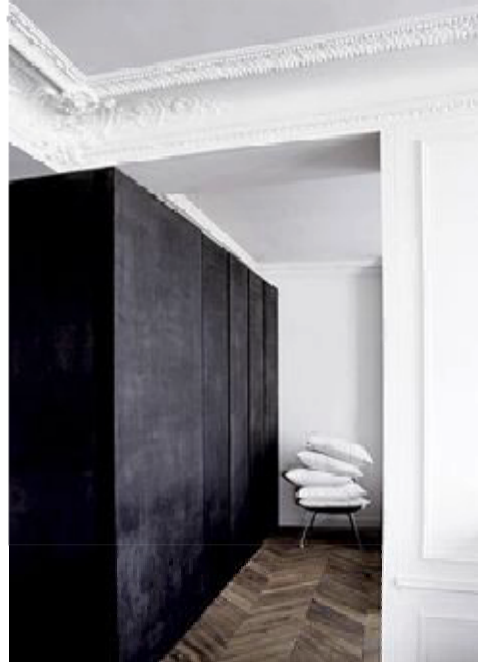
Examples of internal 'pod' treatment (design intent), painted panels (no skirtings), 15mm 'flash-gap' detail at junction with original wall volumes/ party walls and at floors.
