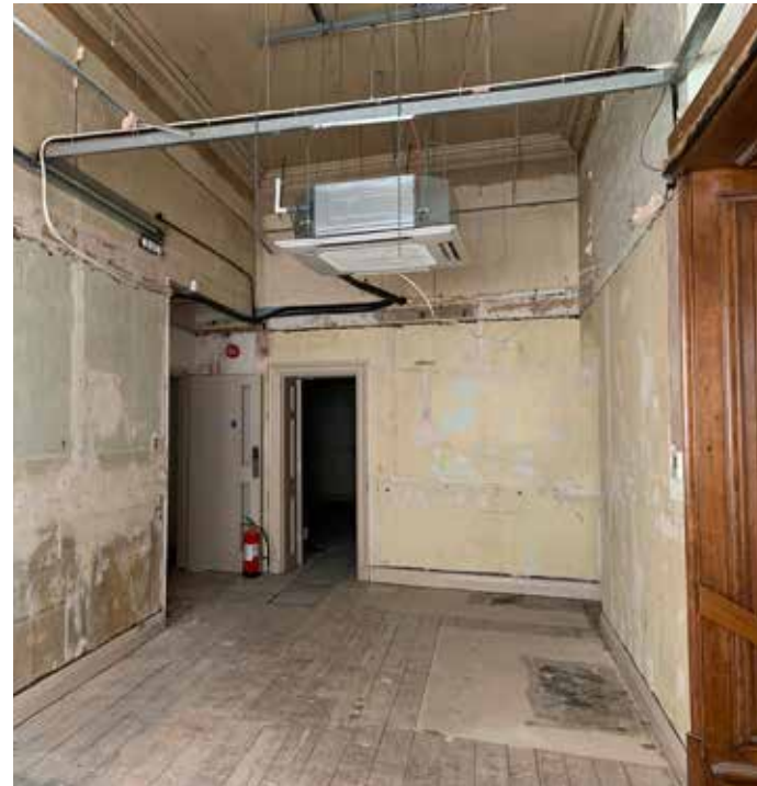
Figure 4.11 The removal of the modern dropped ceiling has reinstated the original volume of the Upper Bank Hall and revealed previously hidden ceiling corning.
