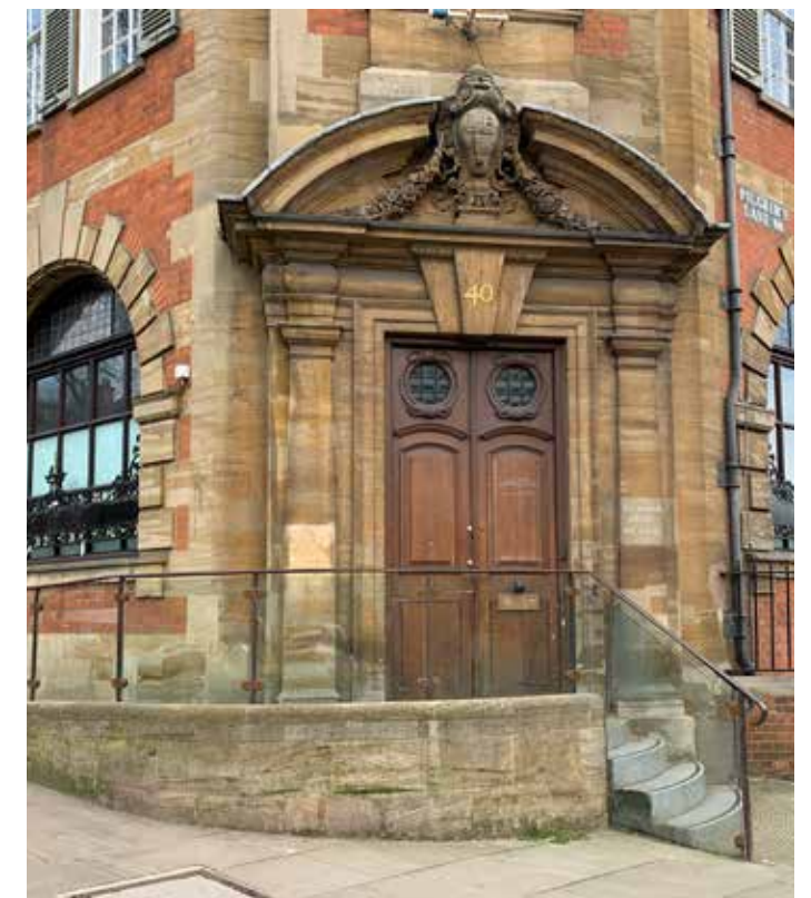
Figure 4.3 The stone doorcase with modern disabled ramp, installed in 2004 following Listed Building Consent. Stonework to the left of the arched pediment presents evidence of a former sign
