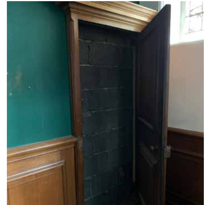
Figure 4.10 Visible cinder block within the infilled entrance between the Waiting Room and Manager's flat detracts from the aesthetic value of the room.
