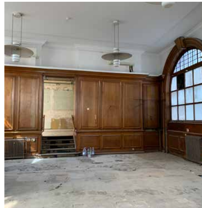
Figure 4.6 Modern carpet has been lifted to reveal a concrete flooring. There is an opportunity to enhance the aesthetic value of the space through improving the quality of modern finishes and making reparations to the panelling.
