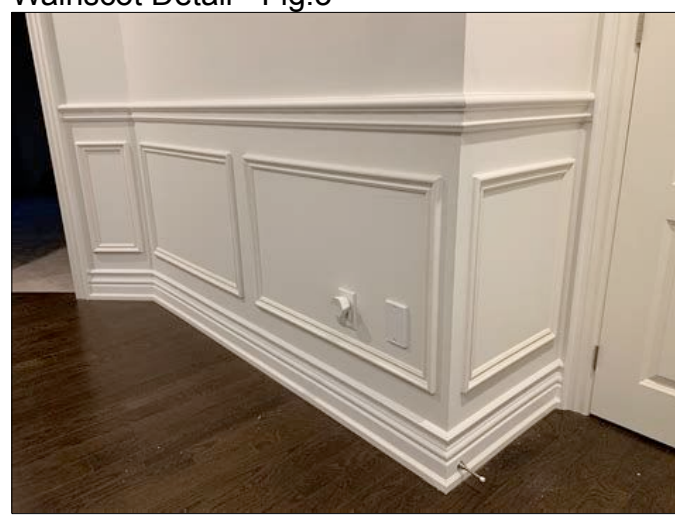
Wainscot - Panelling Detail MDF Moulding & Panel details to create traditional effect wall panelling - Contractor to provide set out detail prior to construction
