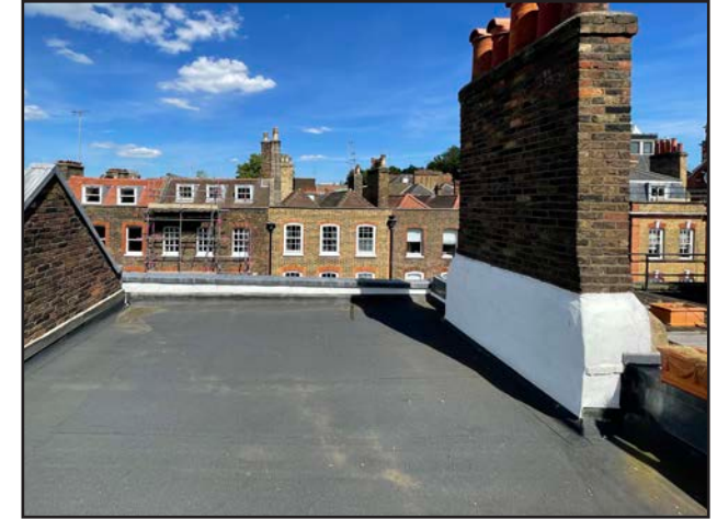
Fig. 7 - Existing flat roof to No. 37
