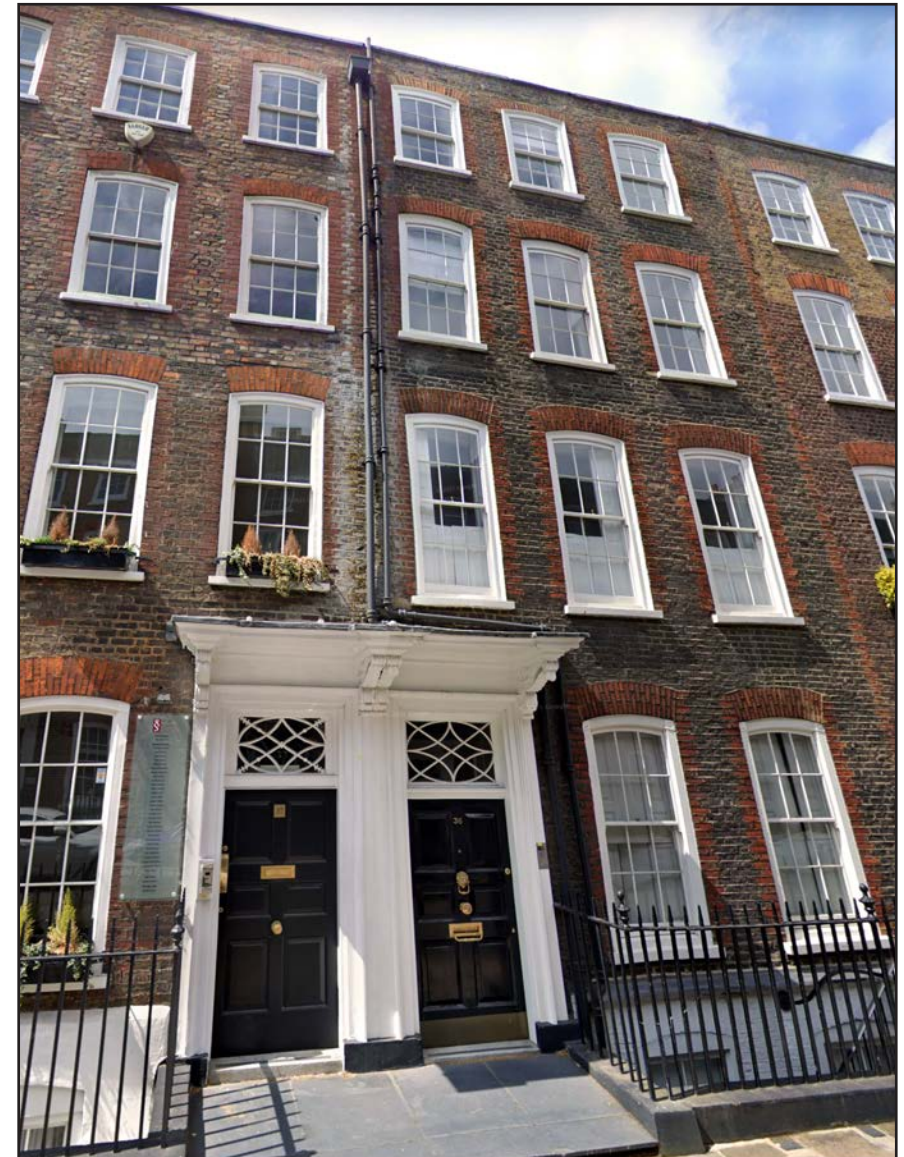
Fig. 1 - Existing shared rain water pipe and soil vent pipe to No.36
