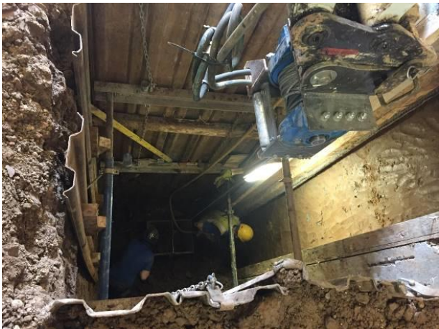
Shored Excavation for an underpin
