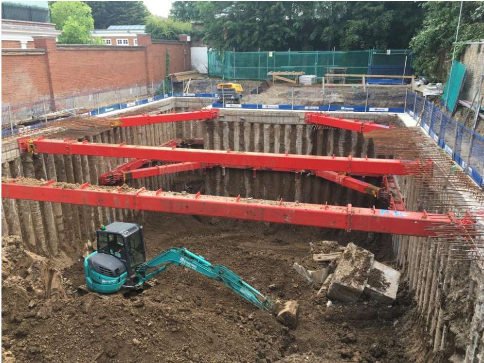
Example of the type of propping that will be necessary during construction and excavation to control and limit ground movement
