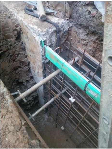
Construction of a Basement Wall by Hit-&Miss Sequence
