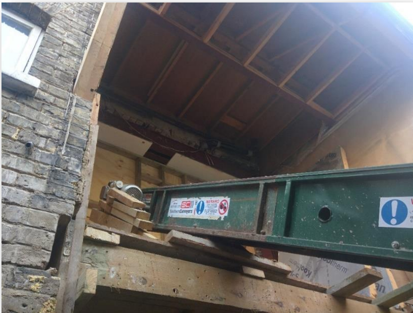
Conveyor to remove arisings
