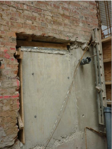
Underpinning To A Masonry Wall
