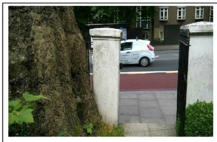
Leaning Gate Pillar - Gate Unable to Close
