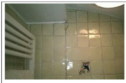
Cracking to Right Hand Wall in Shower Room
