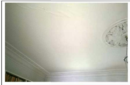
Pulling and Cracking of Kitchen Ceiling
