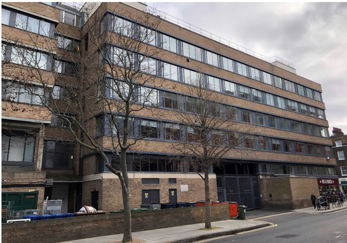
Figure 4 - existing 3m high ground floor extension - right hand side
