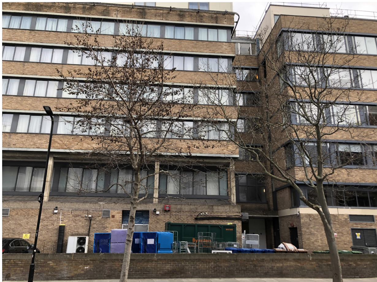
3 REFUSE AREA VIEWED FROM ACROSS HEBRAND STREET NTS
