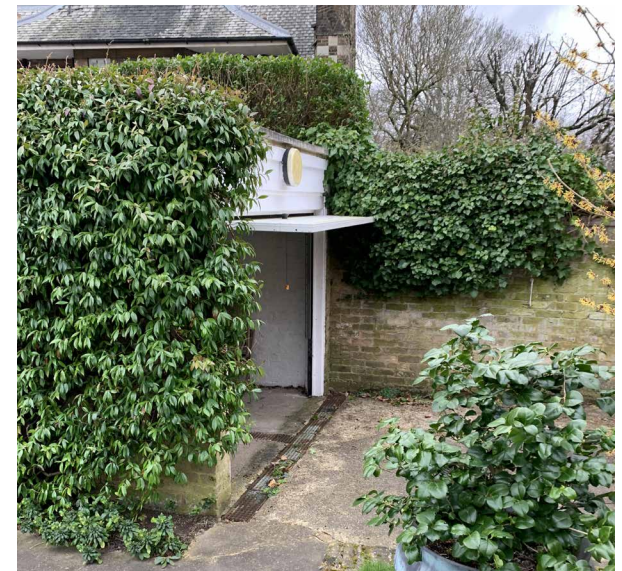
Figure 5. Garage door to be removed.
