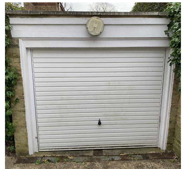
Figure 6. Garage door to be removed.
