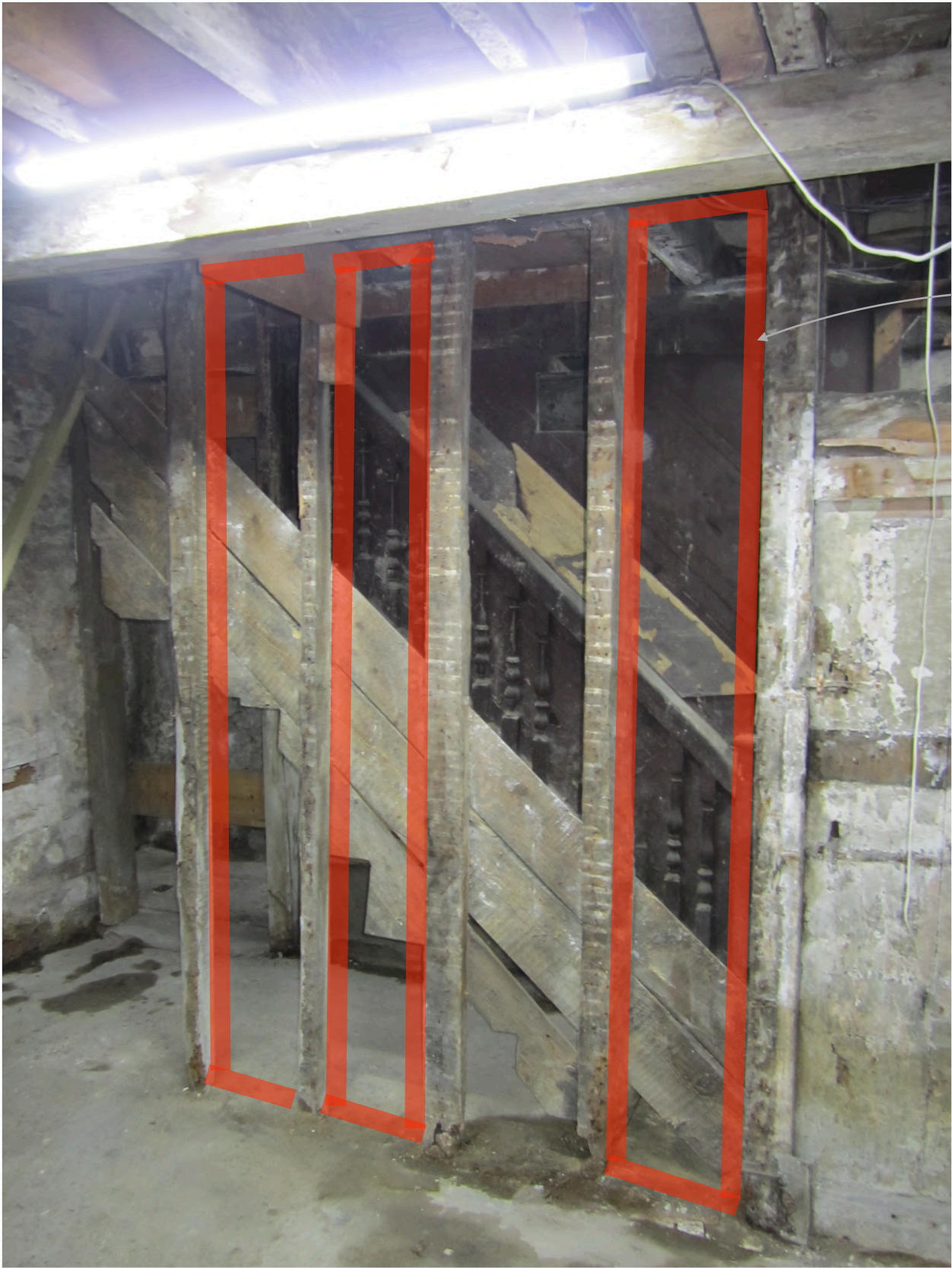
Photo of Stud Wall 'T' with Proposed New Timbers Marked-Over
