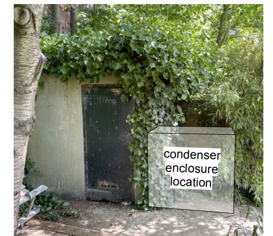
View of Existing Tank Room
