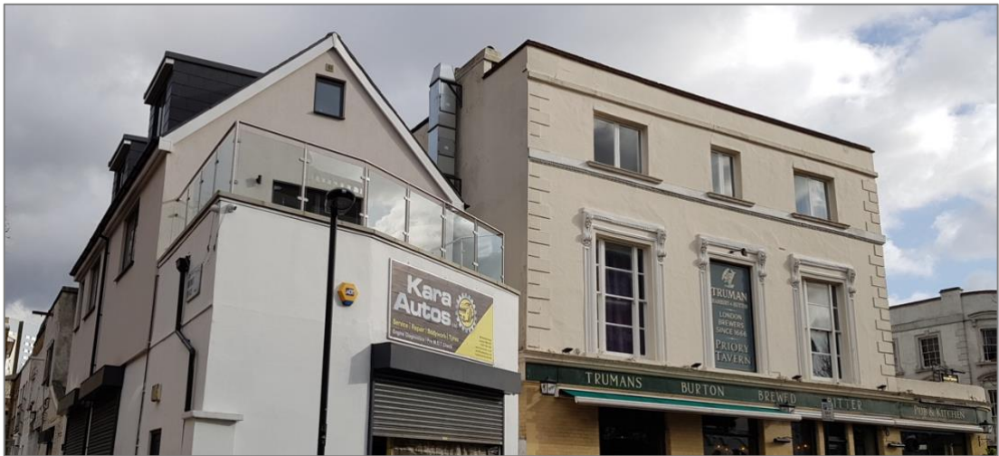
Figure 11: Gable end of Hermit Place showing the addition of a pitched roof with dormer roof extensions and a glazed balcony
