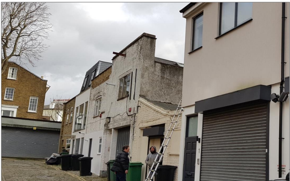
Figure 10: Properties on Hermit Place, note the variety in appearance and different alterations and mansard roof extension
