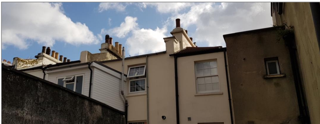
Figure 7: Rear elevation of 246 Belsize Road
