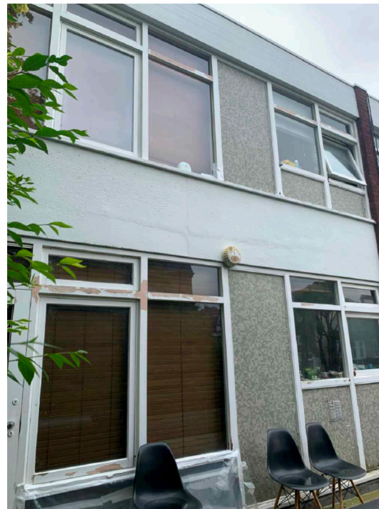
Existing windows showing signs of degradation
