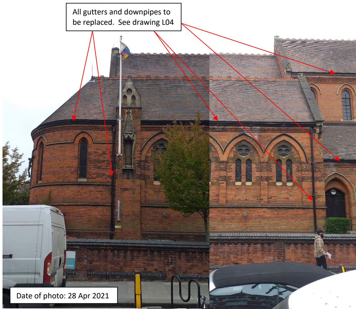
PHOTO 6 (above): North elevation of Chapel. Merged photos
