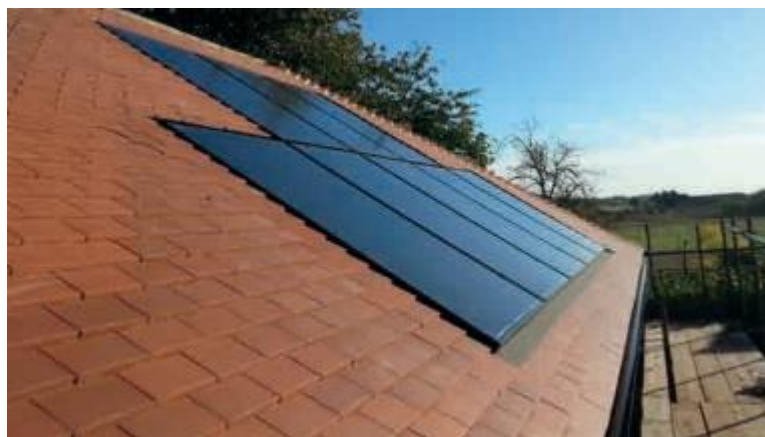
Left: Photo of in-roof system from proposed installer's product literature.
