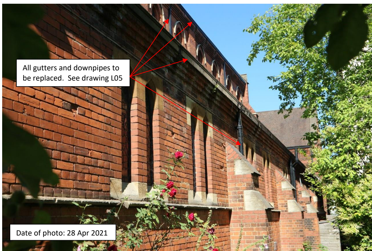
PHOTO 9 (above): South elevation
