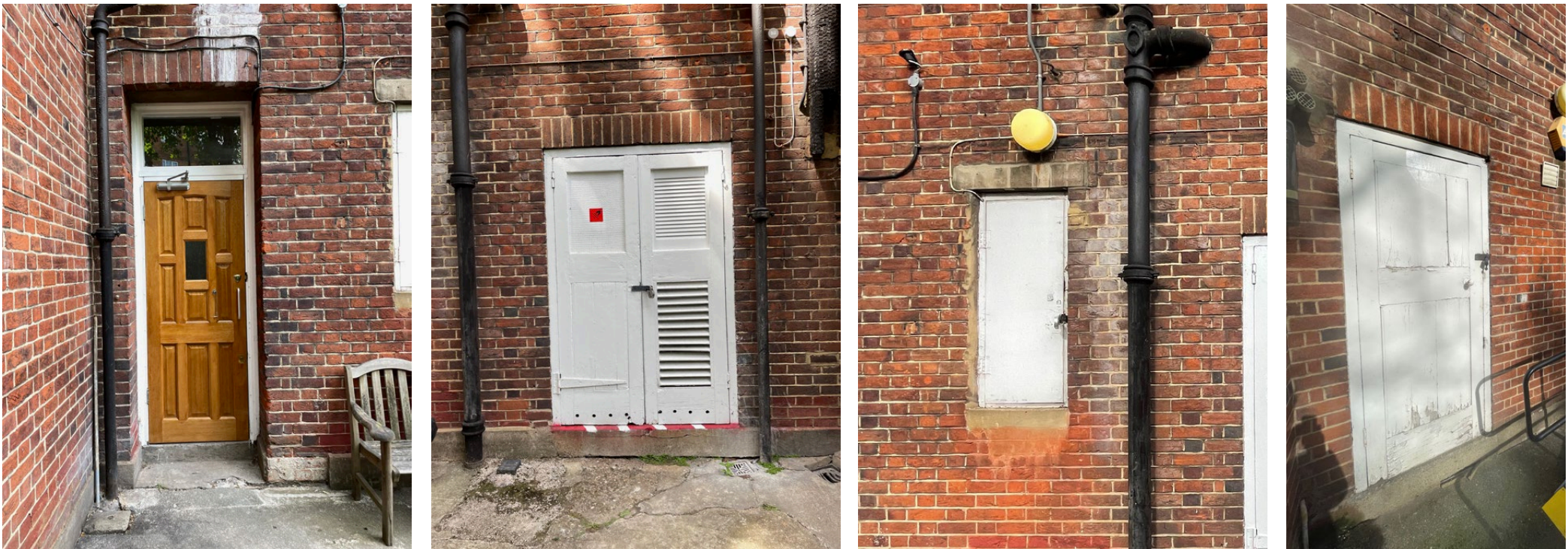
↑ Photos of existing poor quality/defective doors to be replaced
