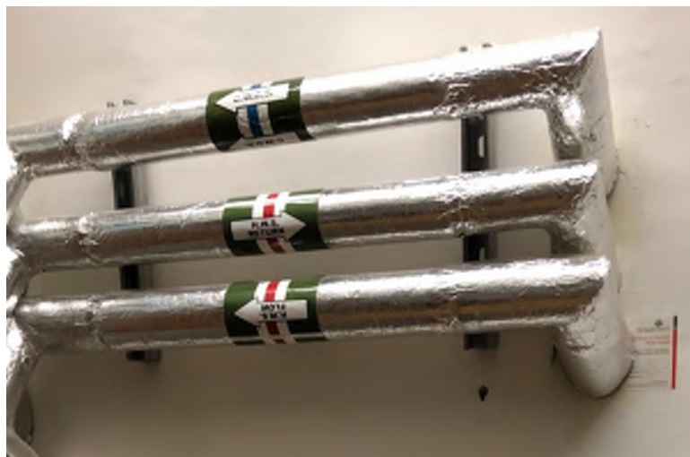
Figure 11 – Typical pipework arrangement with insulation currently installed in the Wilkins Building
