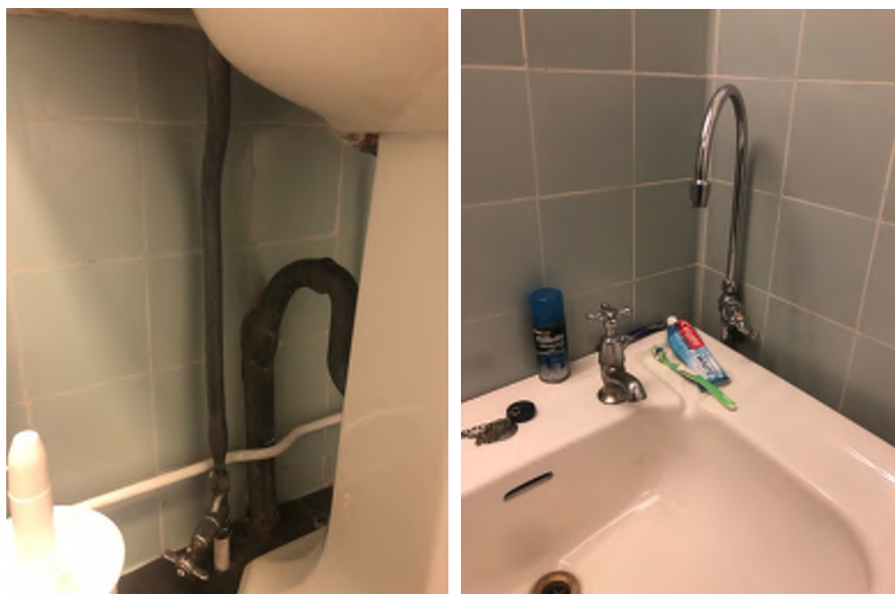
Figure 3 - Lead pipework in Provost's bathroom
