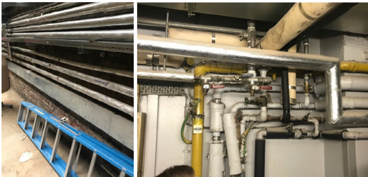
Figure 2 – Examples of complicated piped connections on lower ground level. The picture on the left shows 2 sets of 3 pipe runs (cold, hot flow and return) supplying the same area. The picture on the right shows an example of a numerous branch connections being added over years.
