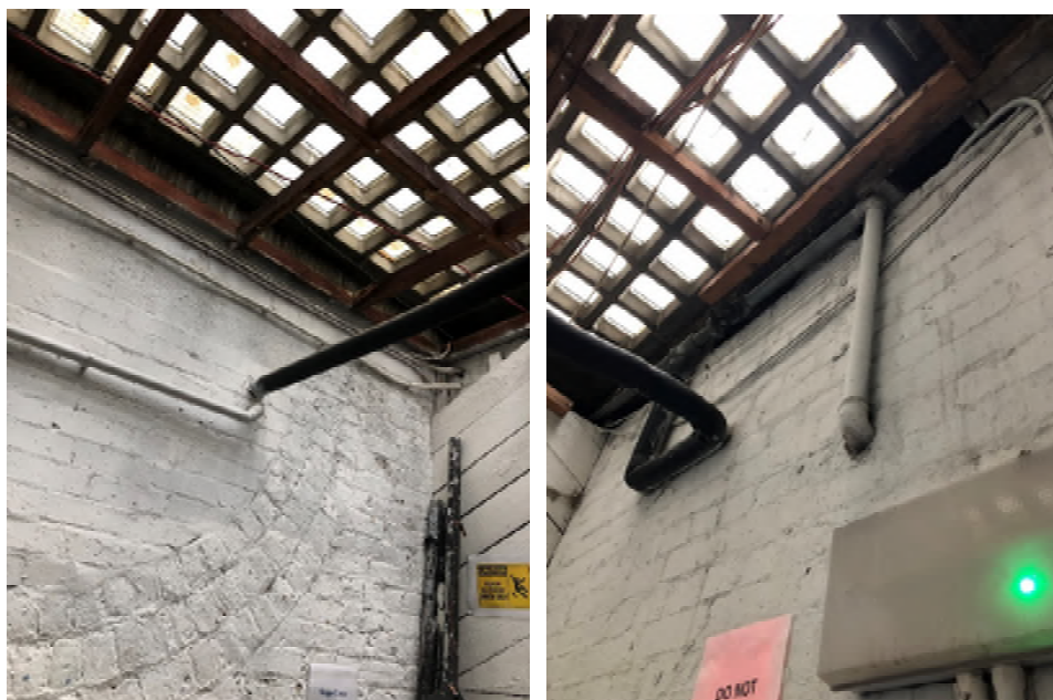
Figure 7 – Existing Mains Water Supply from Gower street
