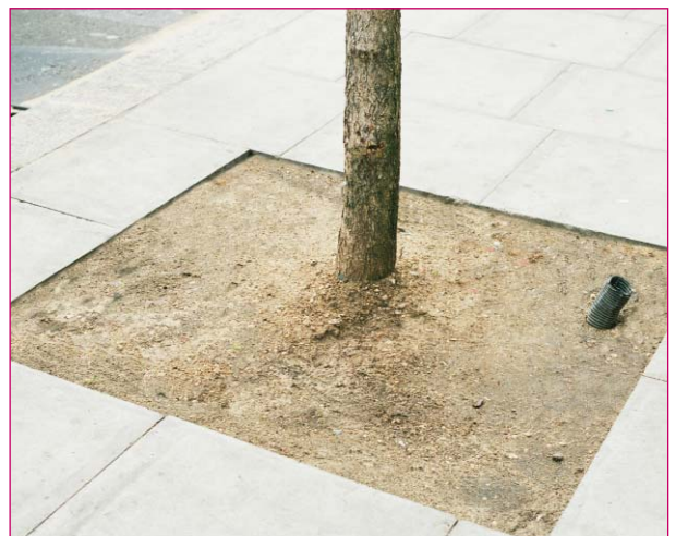
Tree pit in footway with water pipe
