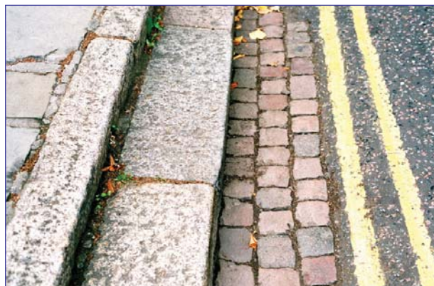
Double granite kerb with drainage channel
