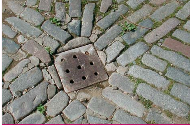
Setts used in traditional drainage techniques
