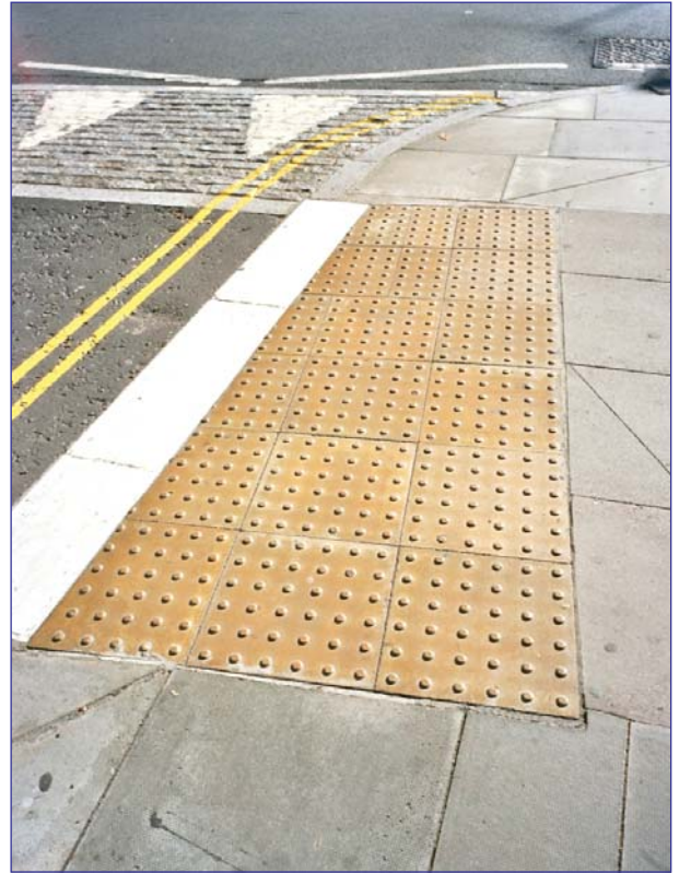
Buff tactile paving at an uncontrolled crossing, on a raised entry treatment
