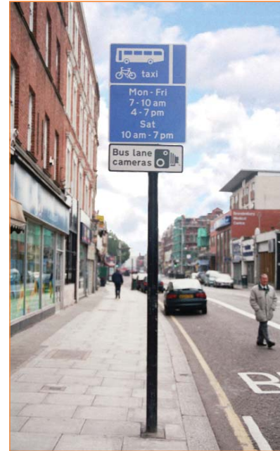
Separated signs carefully aligned on a post
