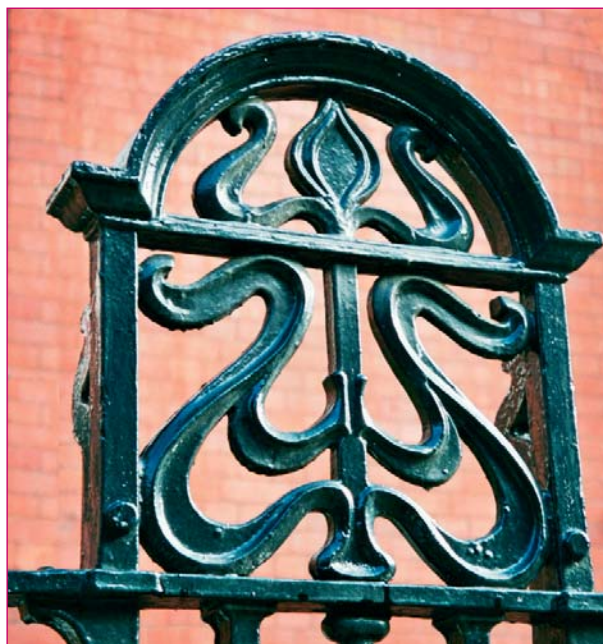
Railings in Bidborough Street
