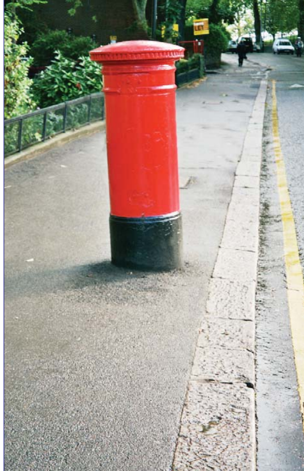
New bituminous footway on Regent's Park Road
