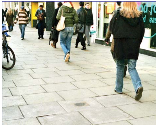
Boulevard paving on a busy commercial street
