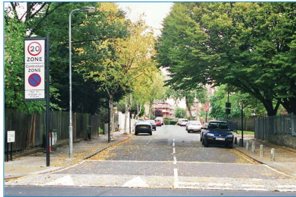
Raised entry treatment in St Cuthberts Road
