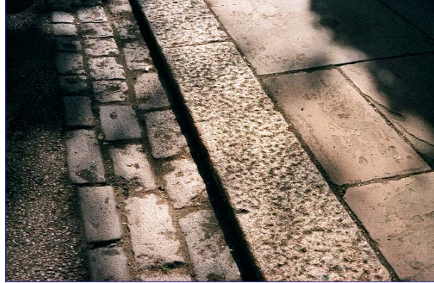
Flat kerb with drainage channel made of granite setts
