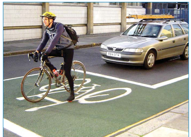
Cycle advanced stop line in Cromer Street
