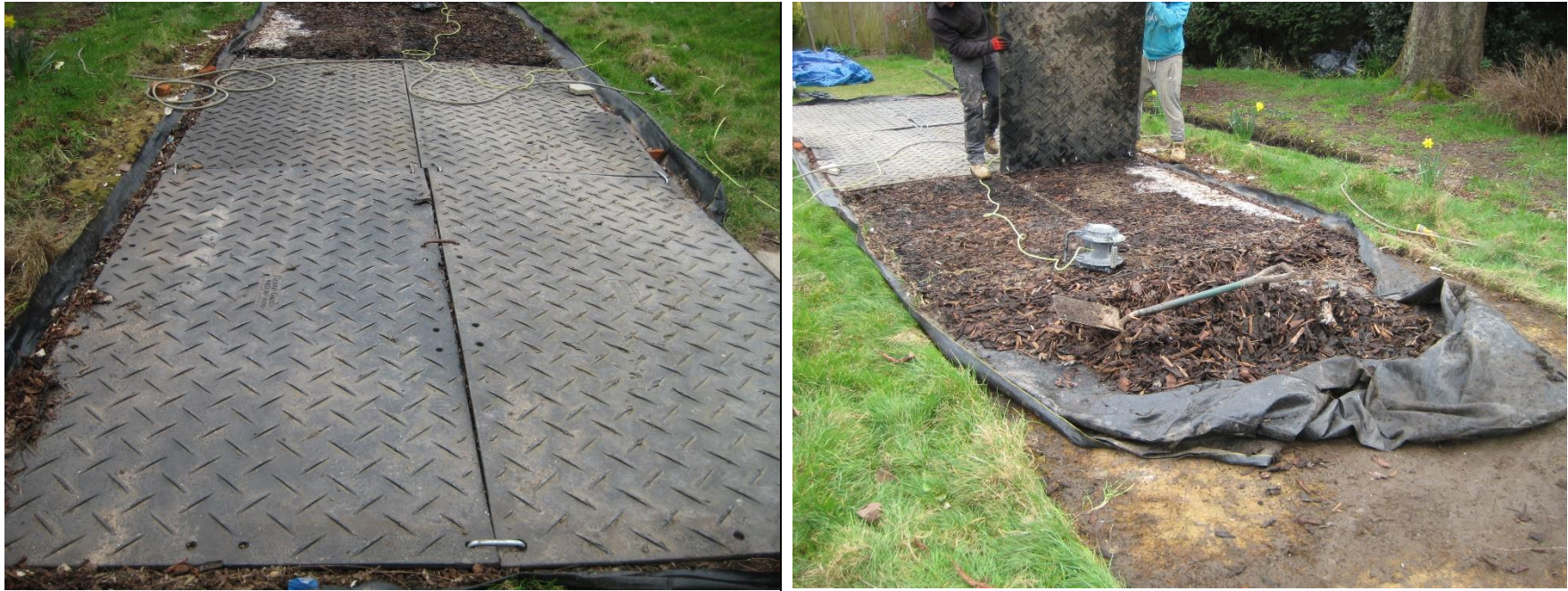
Fig 11 – Temporary ground protection is an effective way of allowing access through the RPA of retained trees. It must be installed prior to any on site activity and maintained for the duration of all works to be effective. Above left Tamla Trees project ground protection in place and above right being removed following the completion of site works. (Note: depending on the length of time it is in place it will adversely affect underlying grass ground cover which will need reseeded/ turfed accordingly)
