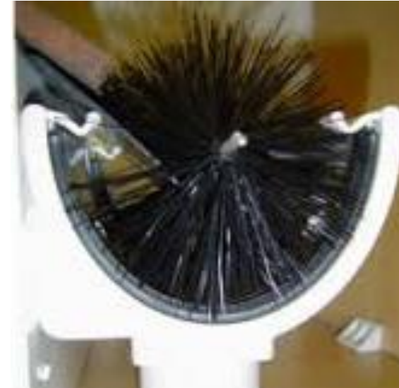
Fig 16 - Suitable gutter guards (2 types shown above) should be fitted to ensure that leaf drop from adjacent trees does not block new guttering leading to potential pressure for tree works.
