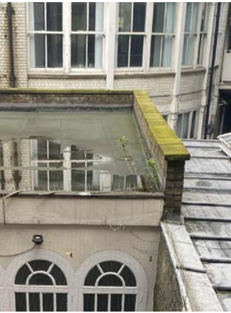
Flat roof coverings pooling
