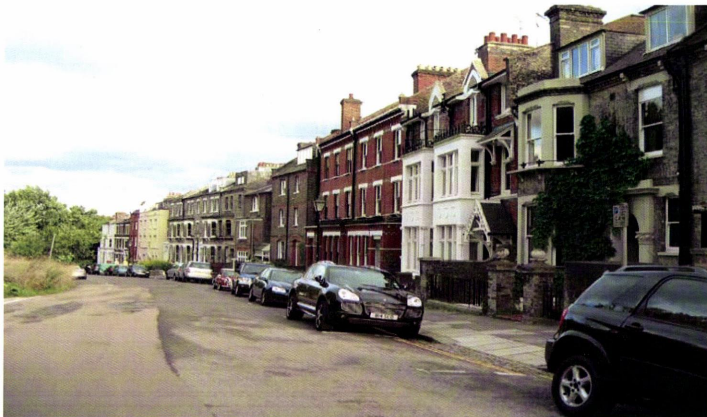
View of the main facade looking down Willow Road
