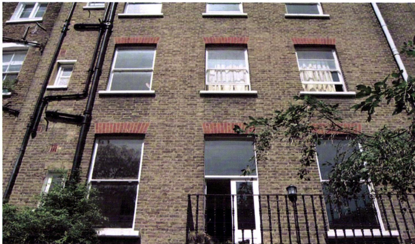
Intermediate part of the rear facade
