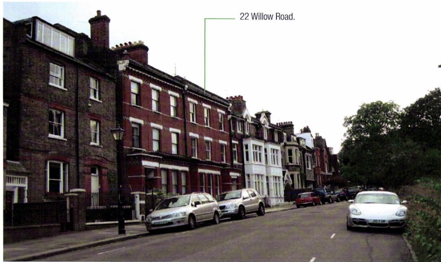
View of the main facade looking up Willow Road
