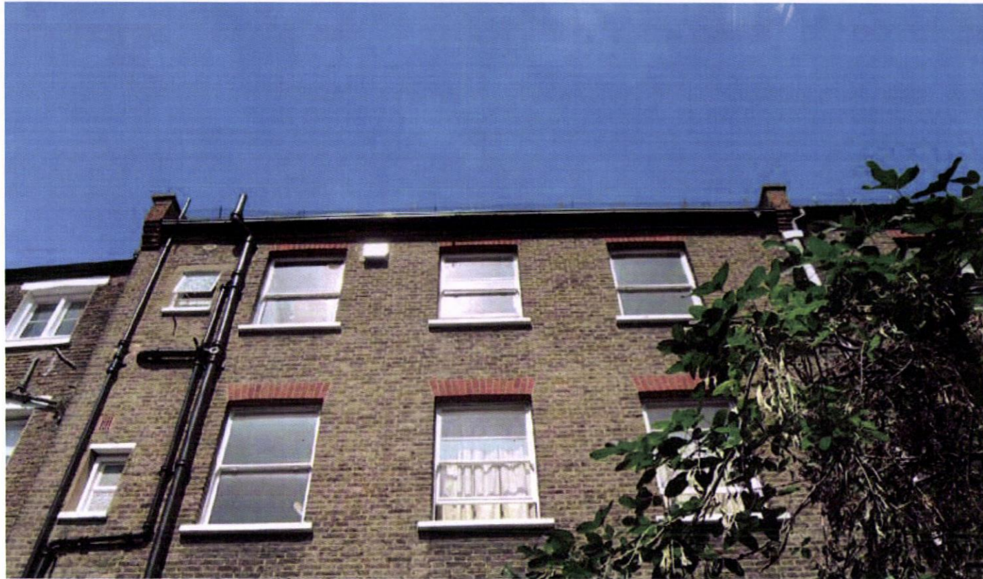
Upper part of the rear facade
