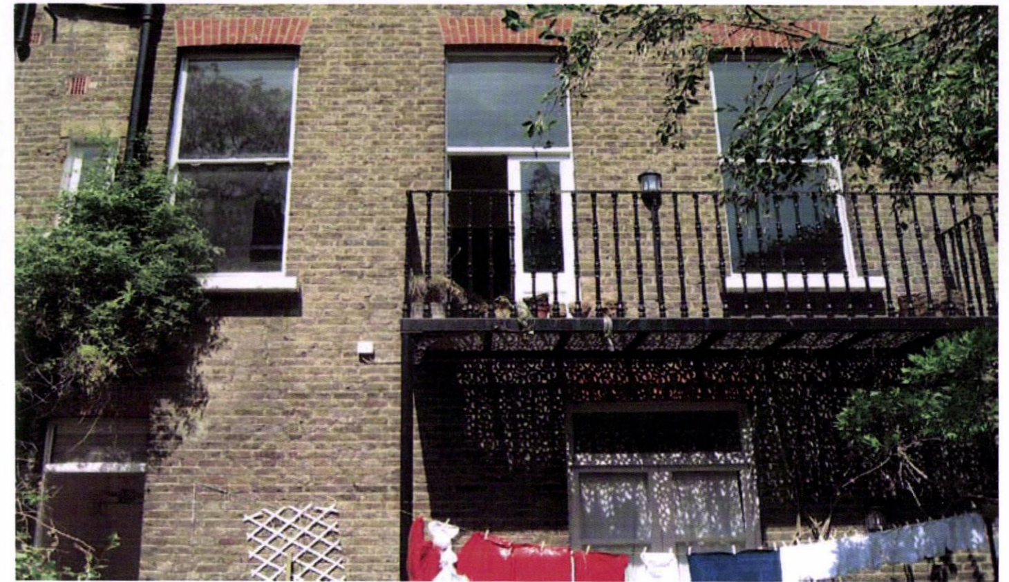
Lower part of the rear facade
