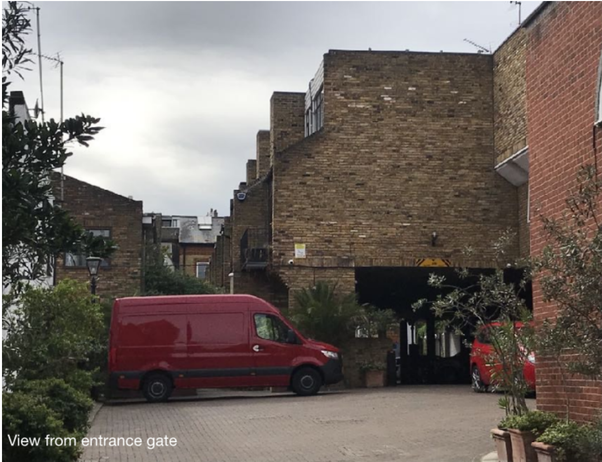
3. View from the entrance gate.
