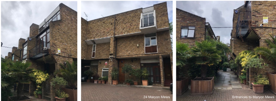
4. Front views of the application sites and terrace row.
