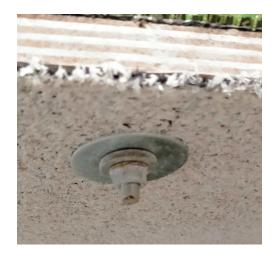
Washers are using on the top and bottom and the Bolts are tightened using a hand drill.
