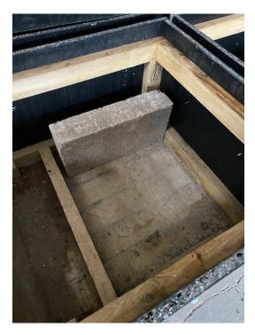
The engineering blocks and/or sand bags are added, totalling 300kg before the lid with the sculpture attached is secured usung 10 x tamperproof screws.
