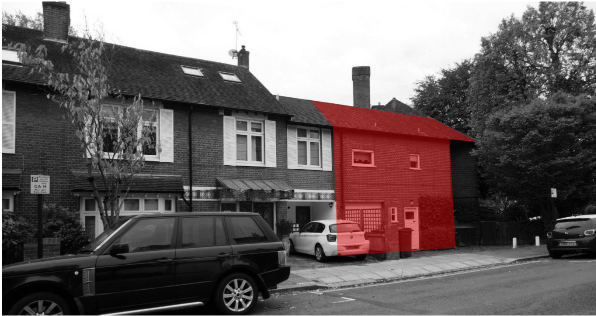
Photo 15: An oblique view of the existing highlighting the way in which it now fills the gap between 12 and 14 Pilgrims Lane.
