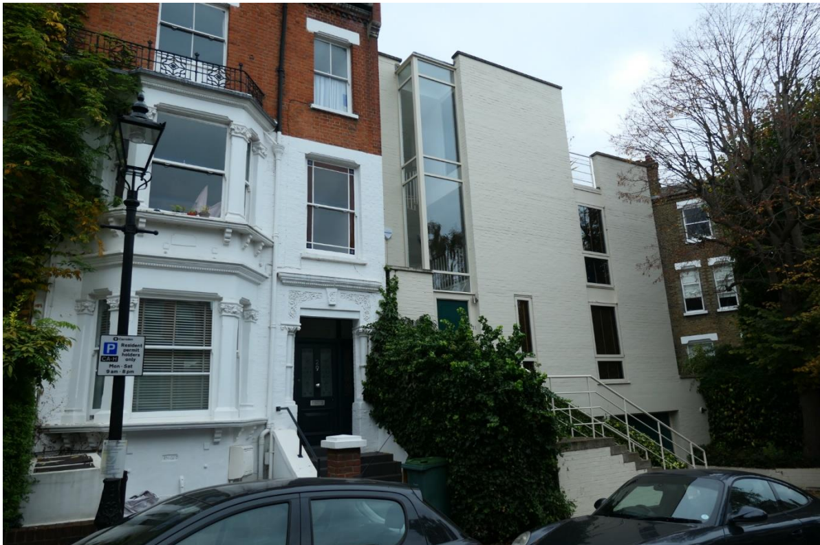
Photo 3: Pilgrim's Lane to the NE - a very modern addition to a late-Victorian house.
