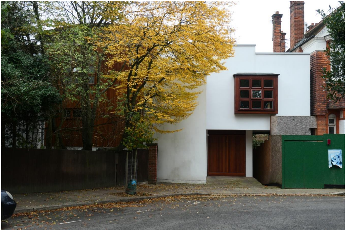
Photo 6: Pilgrim's Lane immediately to the west of the application site – the "1960s building redesigned by SHH Architects in stucco and wood" (as per the Conservation Area Statement).
