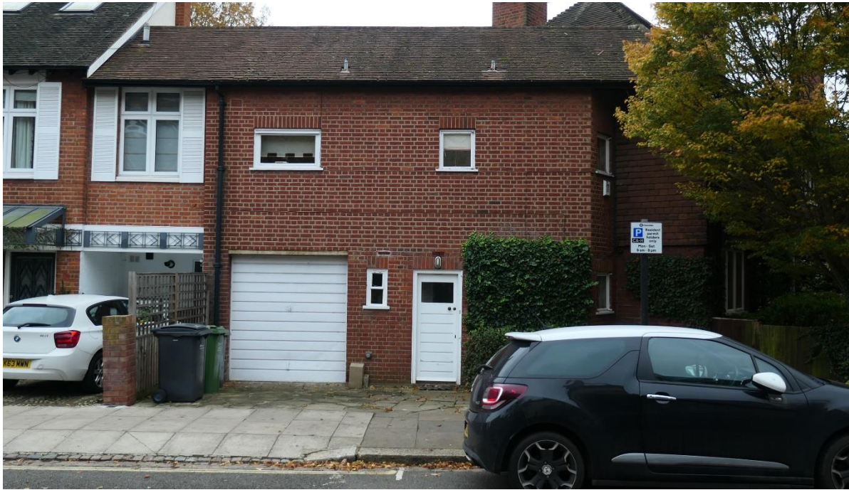
Photo 8: A frontal view of the somewhat awkwardly angled and poorly detailed two storey garage infill structure to the NE of 12 Pilgrim's Lane.
