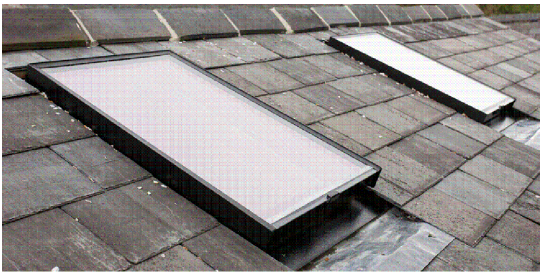
The Conservation Rooflight from The Rooflight Company. Structural opening 720mm x 1350mm approx. Colour: Dark grey (BS00A13). Double glazed. Fixed shut.
