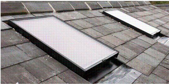
The Conservation Rooflight from The Rooflight Company. Structural opening 720mm x 1850mm approx. Colour: Dark grey (BS00A13). Double glazed. Fixed shut.
