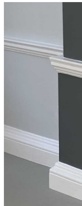
REFERENCE IMAGE Photo of existing skirting and dado detailing on the first floor, both of which are unusually deep. New skirting and dado details have been specified to match
