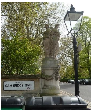
Figure 21 Pier 1 leaning westwards towards the road
