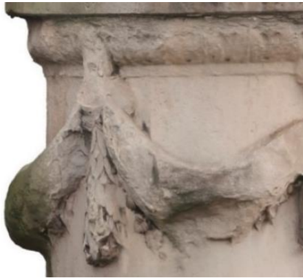
Figure 1 MP2 Almost complete erosion of detail on the swags and the central knot. Small areas survive where protected from the water run-off.
