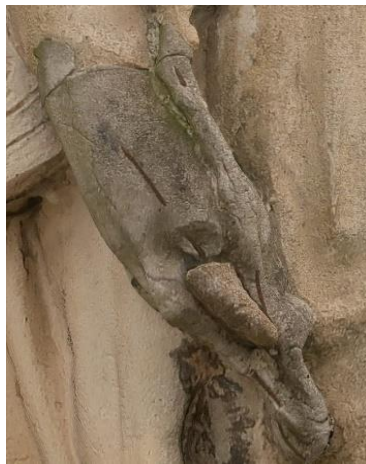
Figure 49 MS3.1. Ferrous armature for the hand associated with repairs
