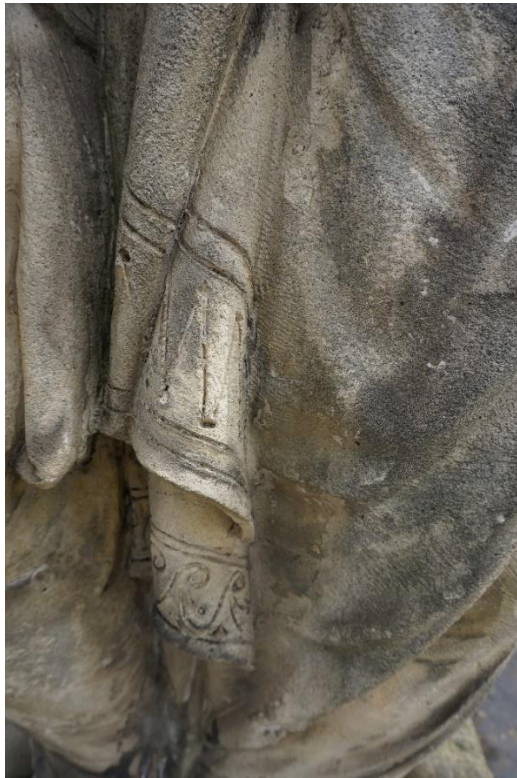
Figure 79 MS2.1 environmental pollution deposit.
