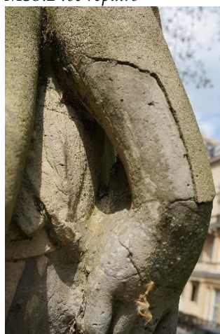
Figure 66 & 67 MS1.2 damage to hand and foliage stalk, also arm repair. Ill-fitting but stable
