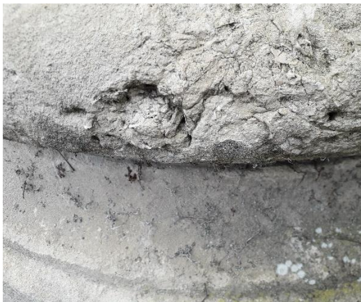
Figure 27 Erosion of material around shell fossils
