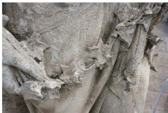
Figure 84 Paint remains in the cracks of applied detail, MS4
