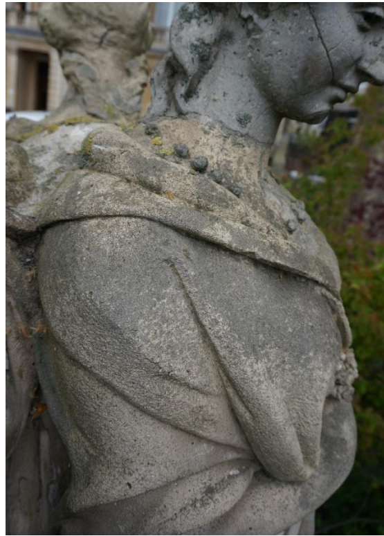
Figure 80 MS1.1 Possibly a mix of dark pollution and biological staining.
