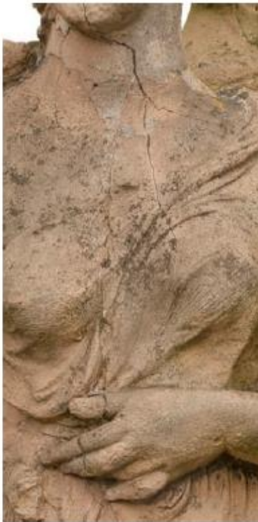
Figure 50 MS3.1 crack running from head through torso ad fingers
