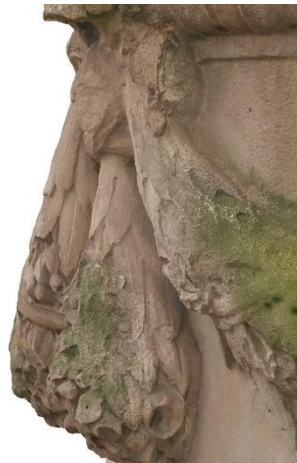
Figure 39 MP1 areas of spalling and loss
