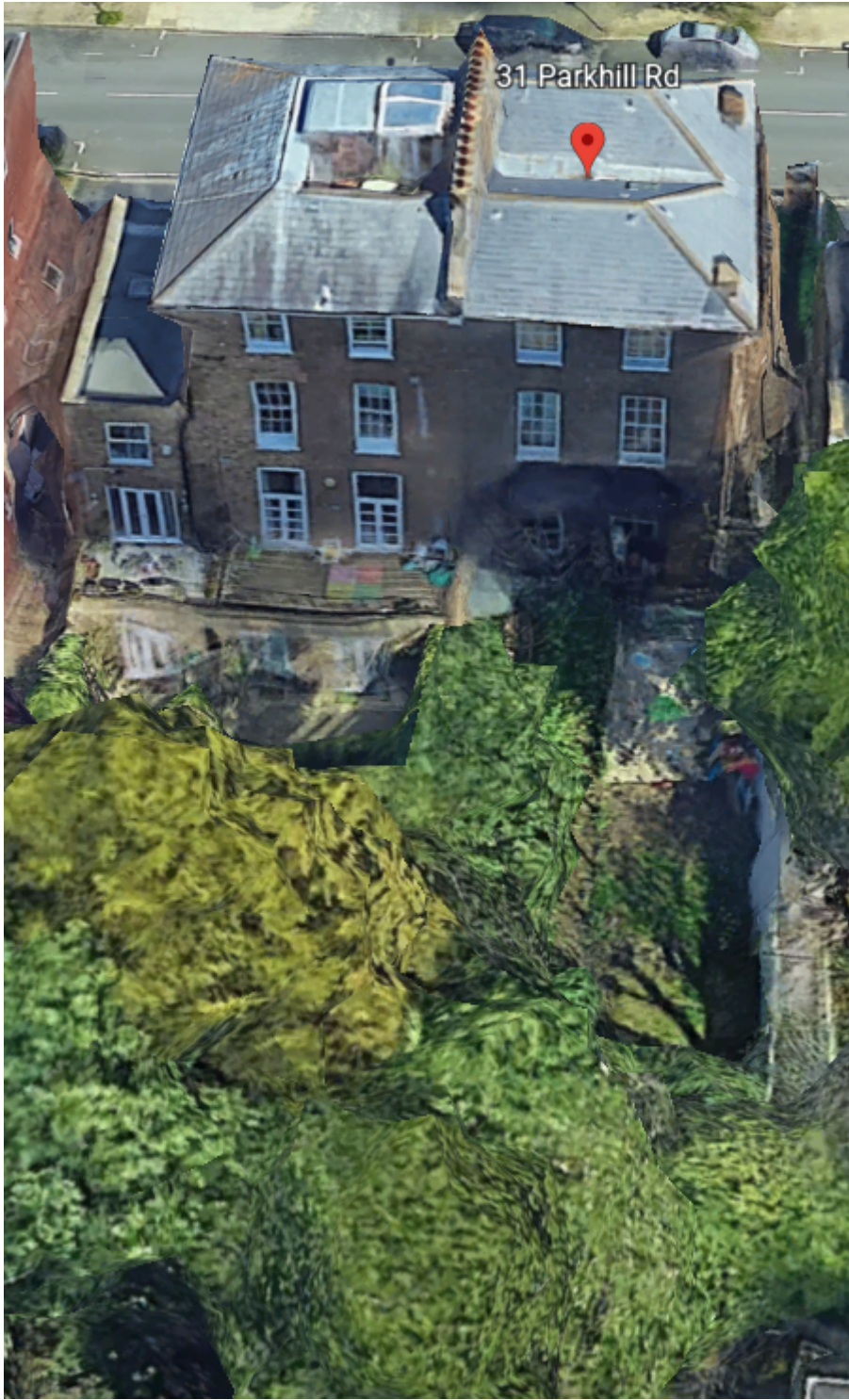
2. Aerial view of rear elevation and rear garden
