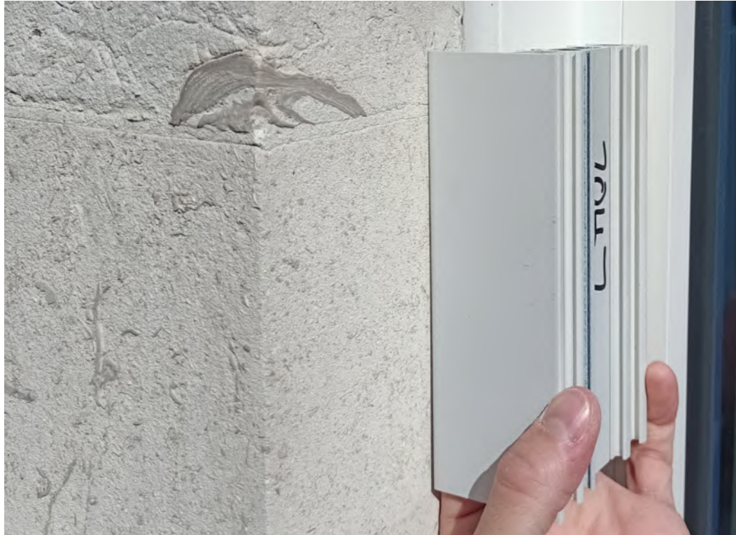
RAL 7047 against existing stone surrounds
