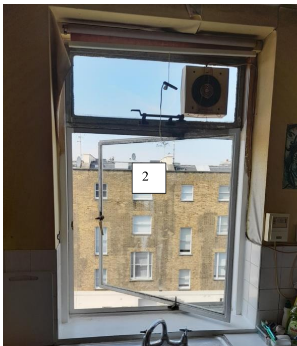
Window 2 Kitchen - ALL WINDOWS OVERLOOK THE REAR OF CHESTER TERRACE
