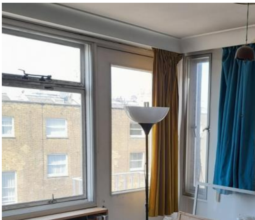
Lounge single door and small return window.
