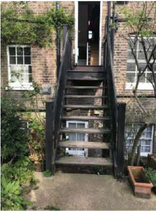
Rear timber stairs detail
