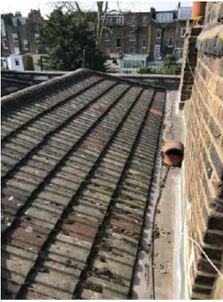
Existing roof pics
