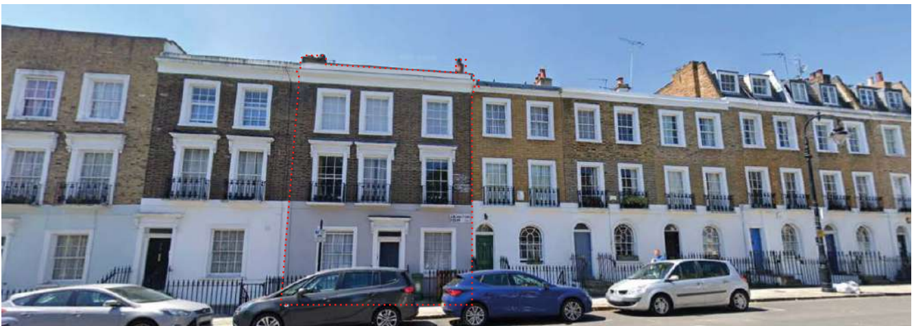
Arlington Road terrace view
