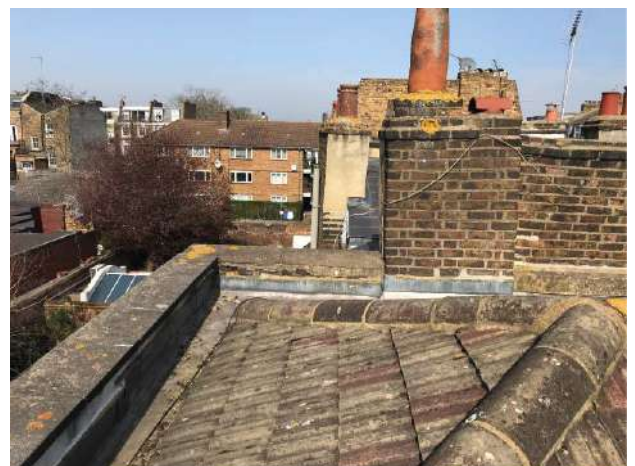
Existing roof pics
