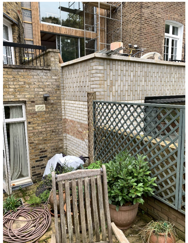
Existing The Side House and 20PR rear extensions
