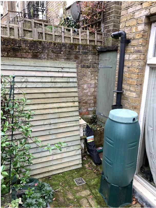
Existing rear patio with No. 18PR
