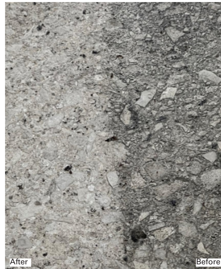
Fig. 2.1.2 Concrete surface before and after cleaning
