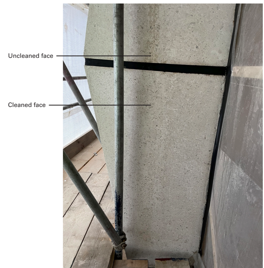
Fig. 2.1.8 Results from second application of Tensid 510 stripper paste
