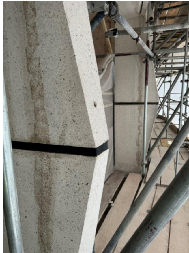
Fig. 2.1.6 Example of adhesive residue from asbestos removal
