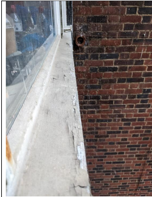
Existing window sill_ weathered and damaged
