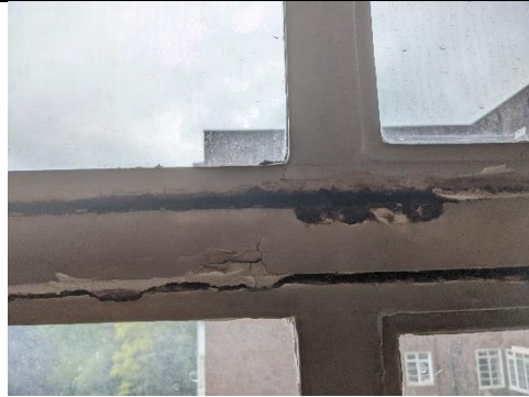
Existing window sill_ weathered and damaged
