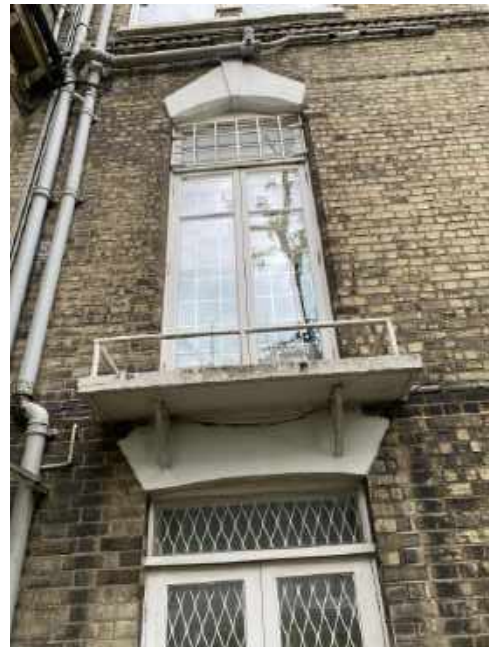
Image 6 – flat 3 projecting window cill
