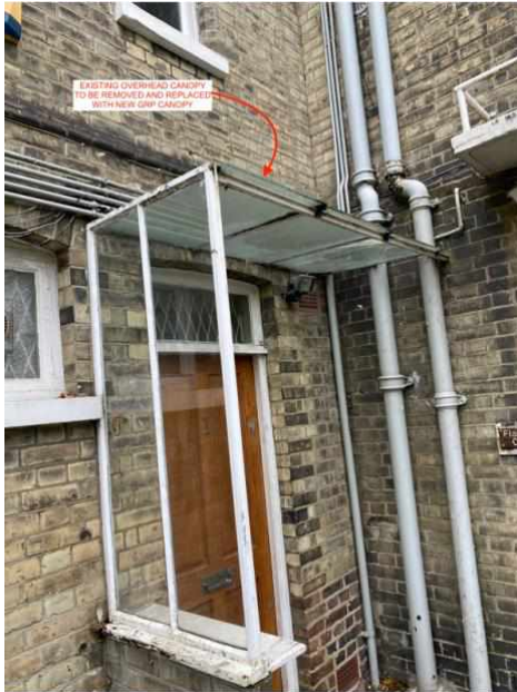
Image 3 – glass canopy to be removed
