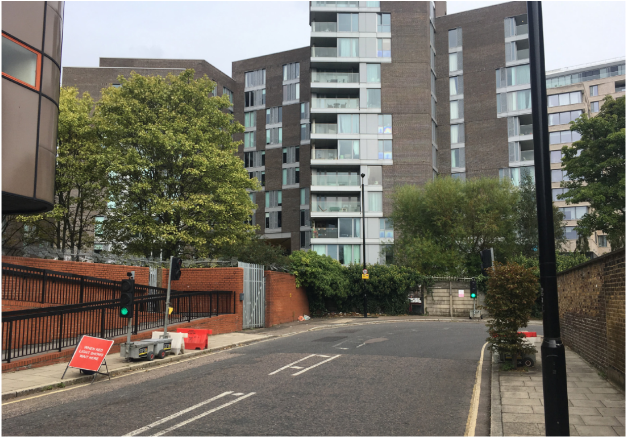
The existing view of the where the bridge steps are proposed to approach Granary Street
