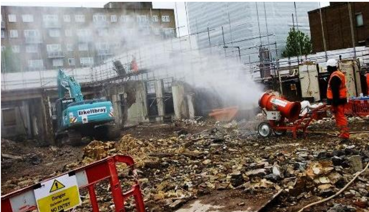
Figure 7: Dust suppression using dust suppressing water machines
