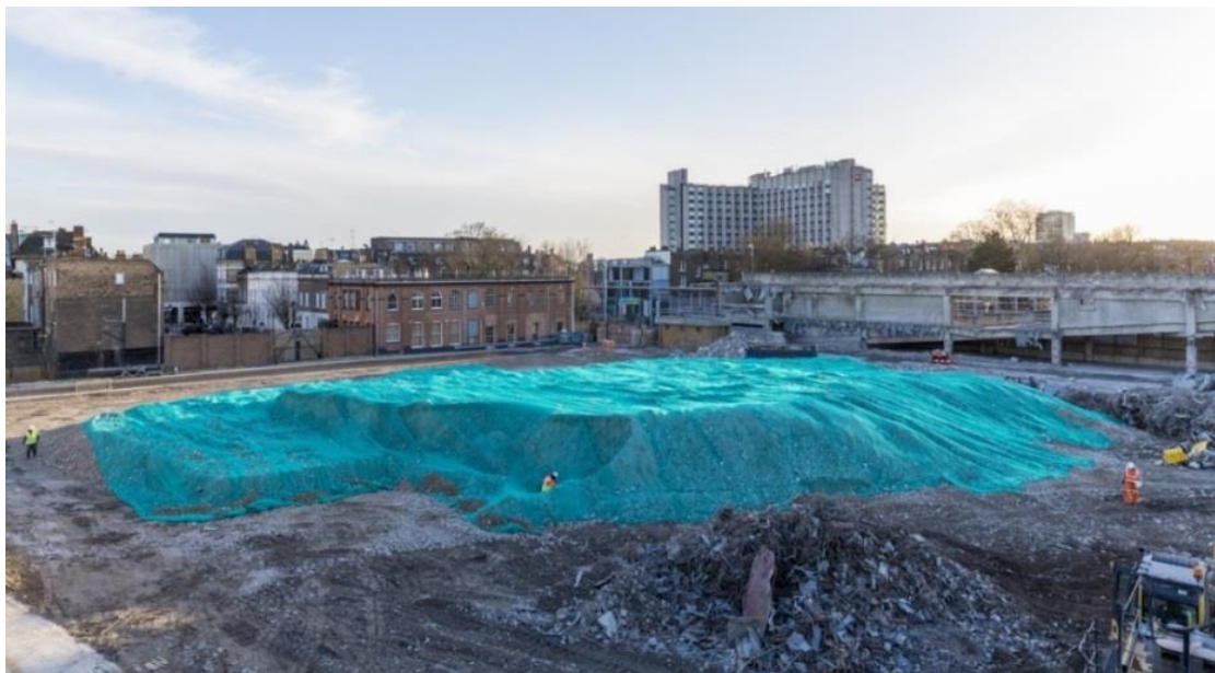
Figure 6: Sheetting of spoil heaps
