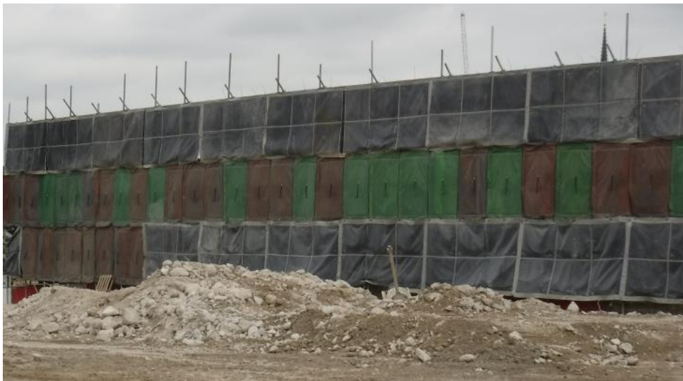
Figure 4: Scaffold with acoustic screens
