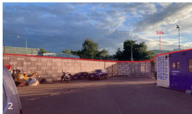
Looking South from the middle of the site.
