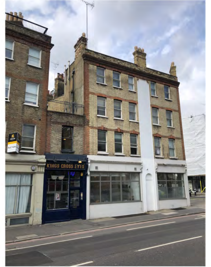
VIEW OF PARTY WALL WITH No.101B KINGS CROSS ROAD
