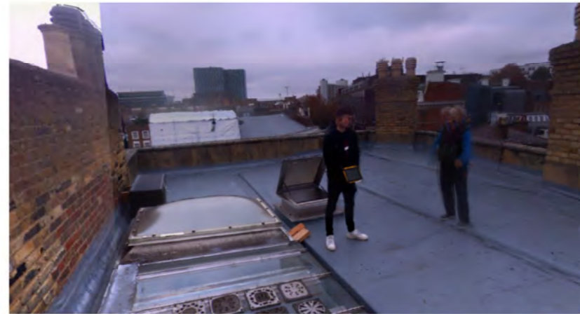
VIEW OF EXISTING ROOF
