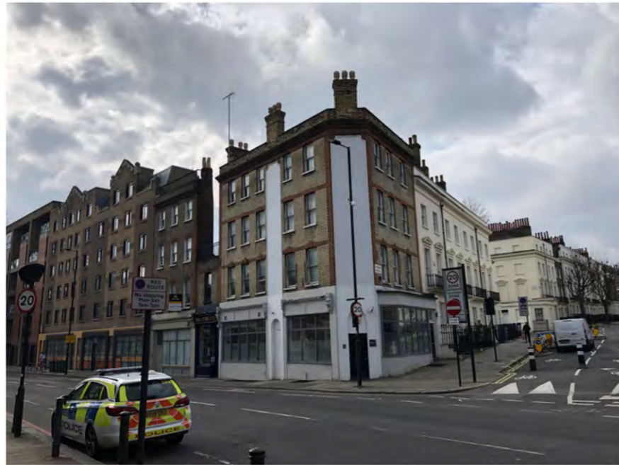
KING CROSS ROAD / FREDERICK JUNCTION
