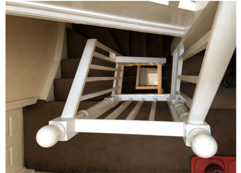
VIEW DOWN EXISTING COMMON PARTS STAIRCASE
