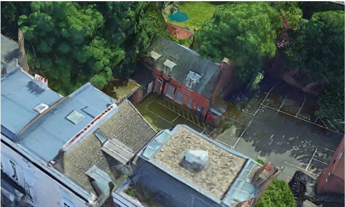
2. Closer-up aerial view of the Stables building
