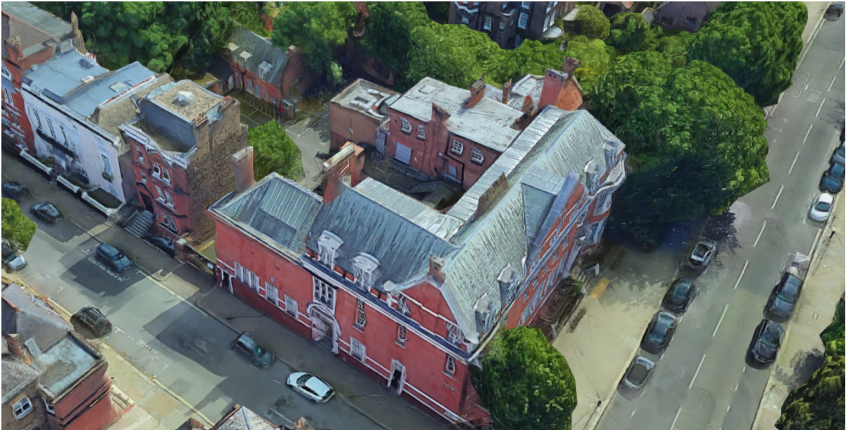
1. Aerial view of the Stables building at the rear of Former Hampstead Police Station, and the access from Downshire Hill
