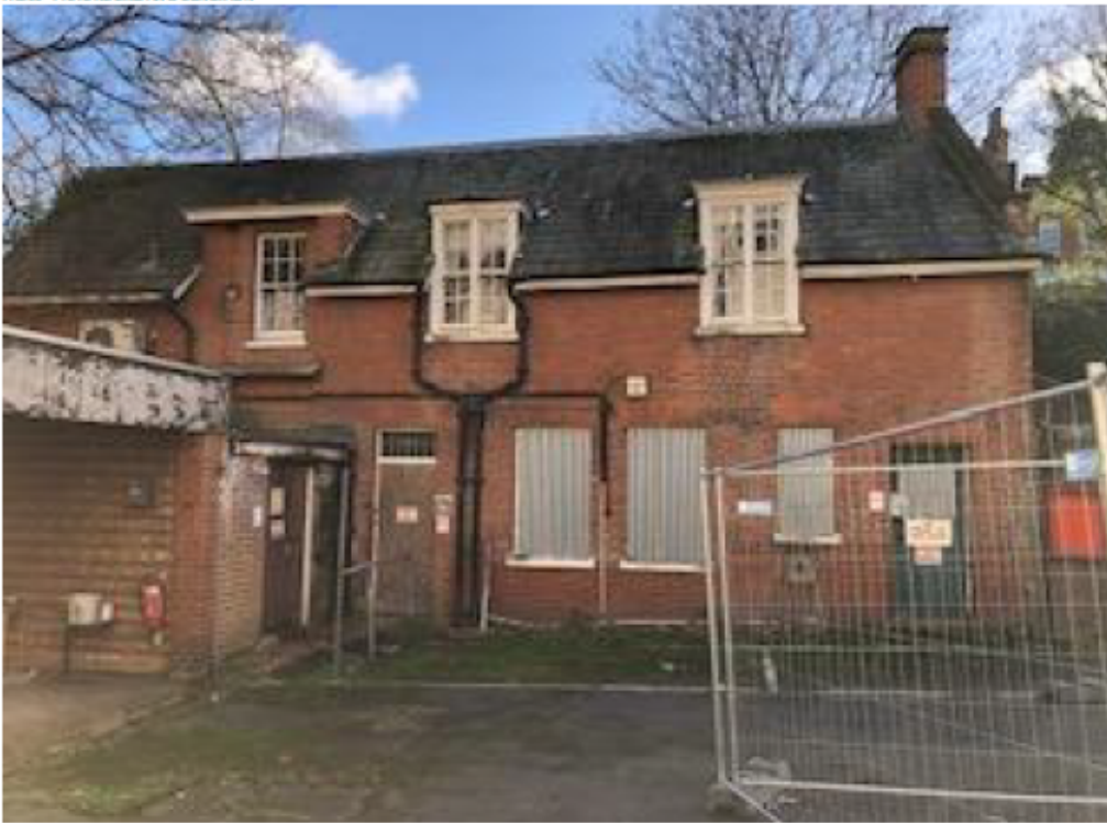
3. The front elevation of the Stables building
