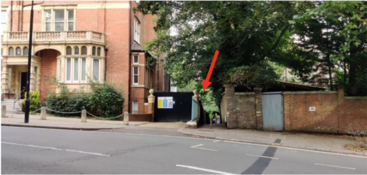
Image 1.01 - Metal fence and stone details to be carefully removed and reinstated at the end of the construction period
